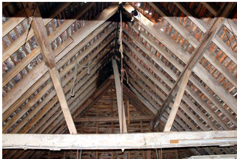
Plate 6: Northern building, roof truss in room G1.
