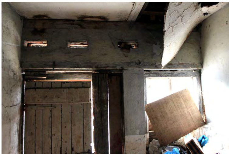
Plate 9: Northern building, ventilation in room G3.
