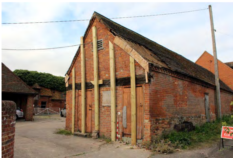
Plate 2: North building, eastern and northern elevations.
