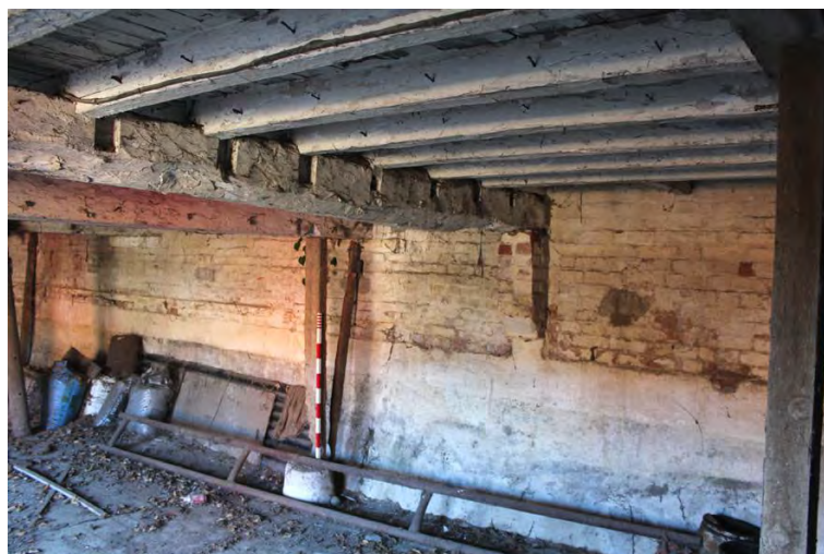
Plate 15: Southern building, room G1 showing reused or repositioned beam.
