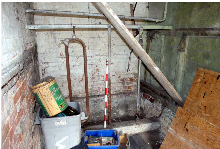
Plate 7: Northern building, trough and collars in room G2.
