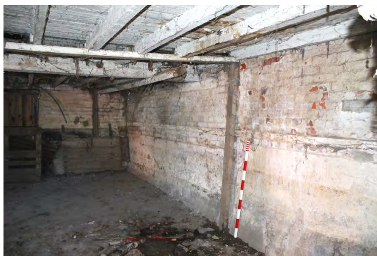
Plate 16: Southern building, southern wall of room G1 showing rail for hay rack attached to ceiling beam and possible partition beam.
