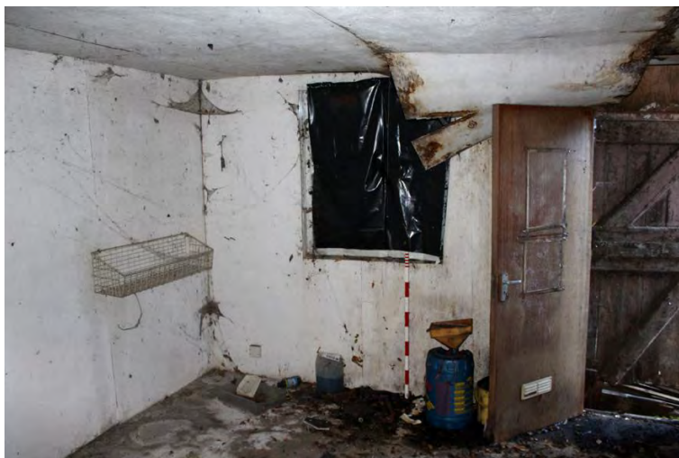
Plate 18: Southern building, northern wall of room G2.
