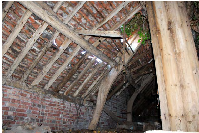
Plate 21: Southern building, roof trusses in room F1.
