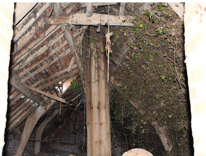
Plate 20: Southern building, roof trusses and vent structure in room F1.
