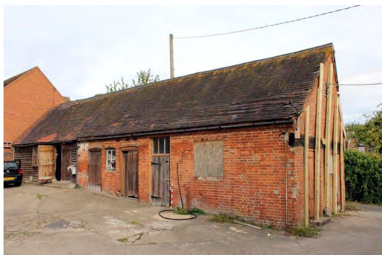
Plate 1: North building, southern elevation.
