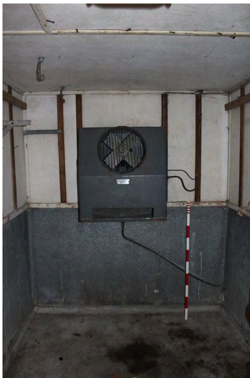
Plate 12: Northern building, western wall of refrigeration room (room G5).
