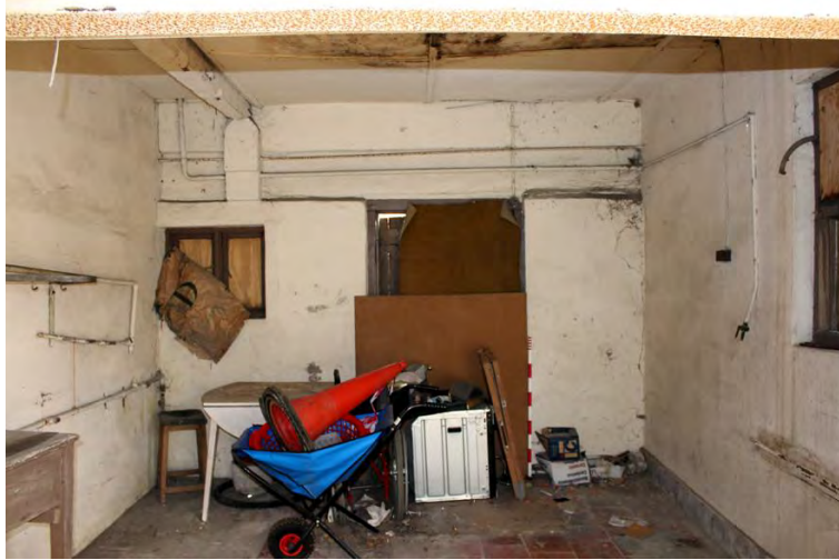
Plate 10: Northern building, eastern wall of room G4b.
