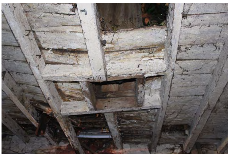
Plate 13: Southern building, square opening in ceiling of room G1.
