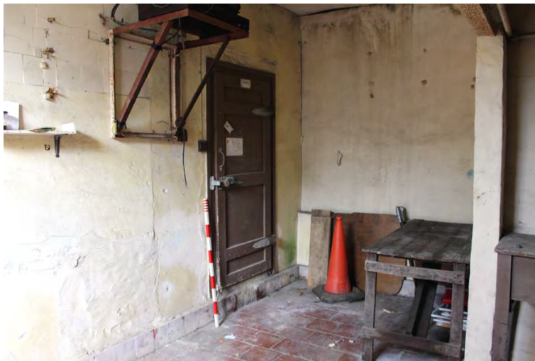
Plate 11: Northern building, room G4a showing later refrigerator door.
