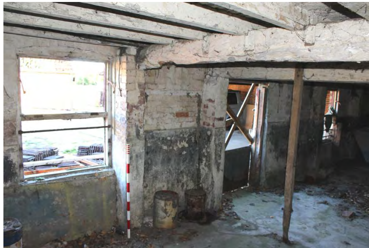
Plate 14: Southern building, northern wall of room G1
