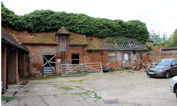
Plate 3: Southern building, northern elevation.
