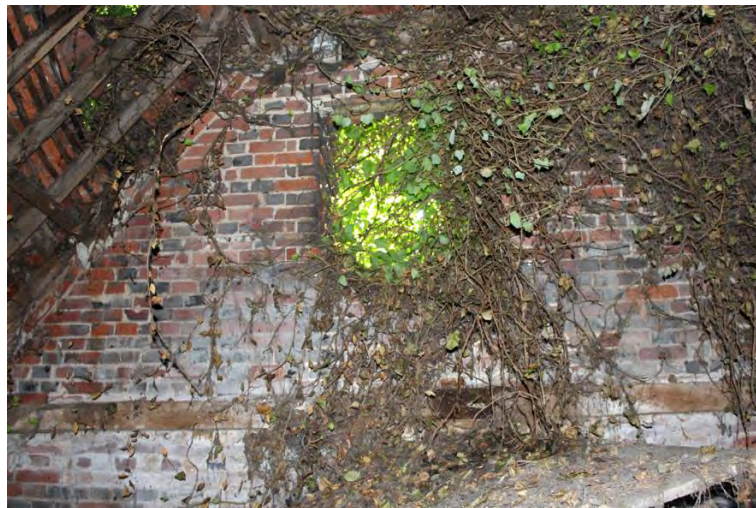
Plate 22: Southern building, window in eastern gable wall in room F1.
