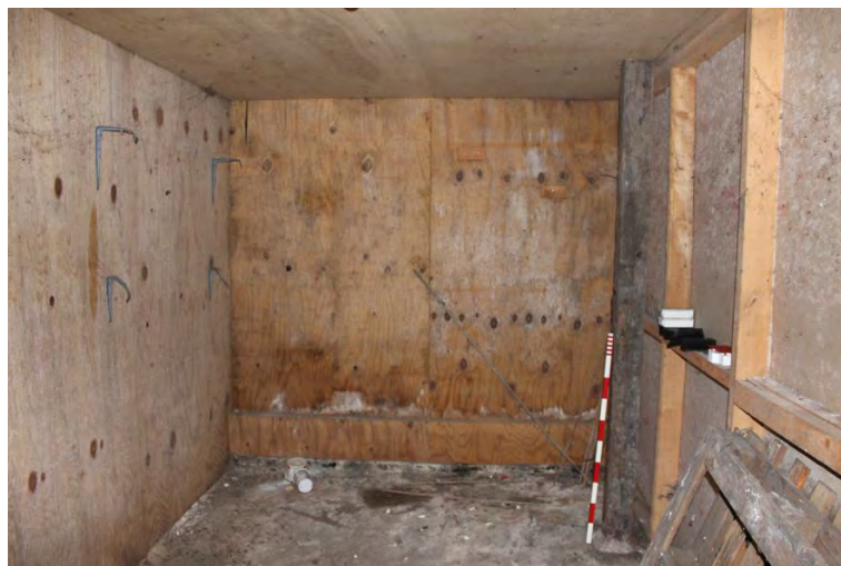
Plate 19: Southern building, southern wall of room G3.
