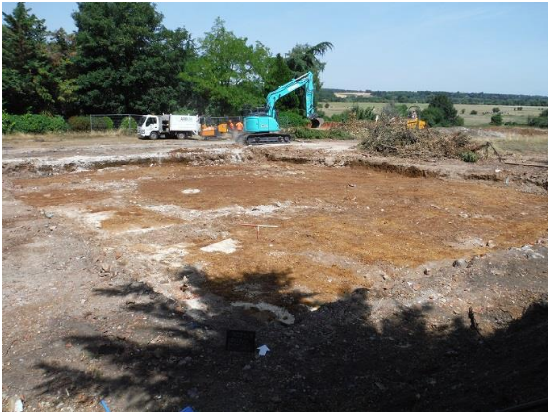
Plate 2: Central Basement Area Stripped Down To Natural Horizon.
