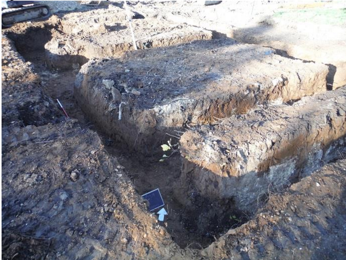
Plate 1: North-East Area of Footings, Looking North.
