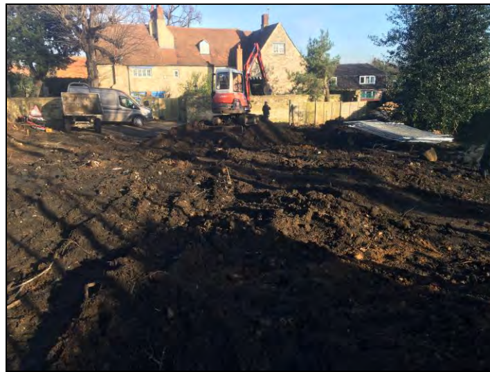
Plate 1: North facing view of the levelled site from the south end
