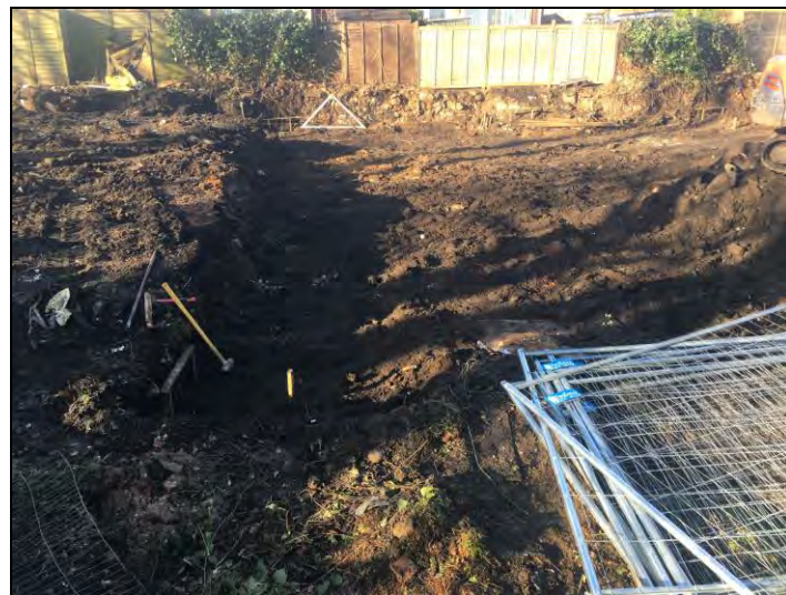
Plate 2: West facing view of the reduced construction area
