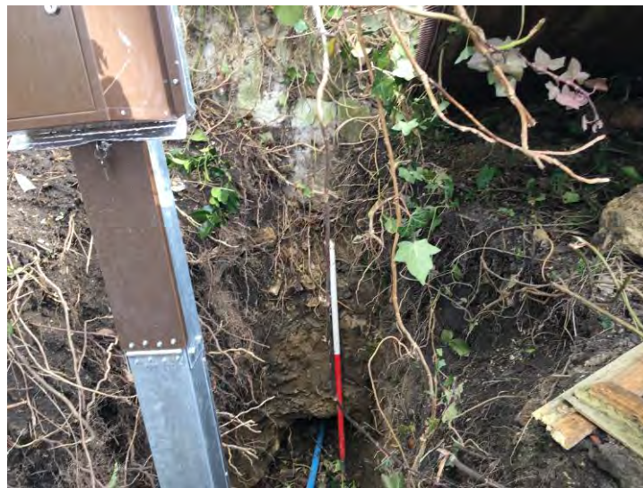
Plate 6: West facing section of cable duct
