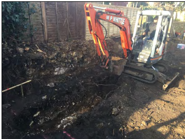
Plate 3: North-West facing view of initial trenching
