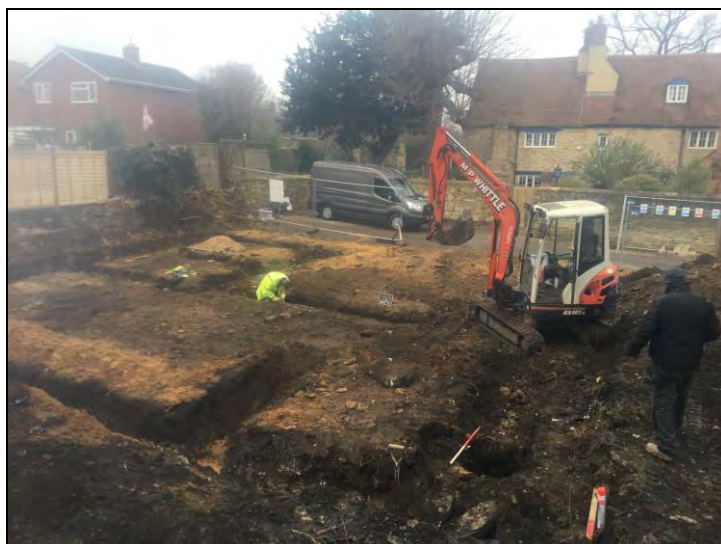
Plate 4: North-West facing view of site
