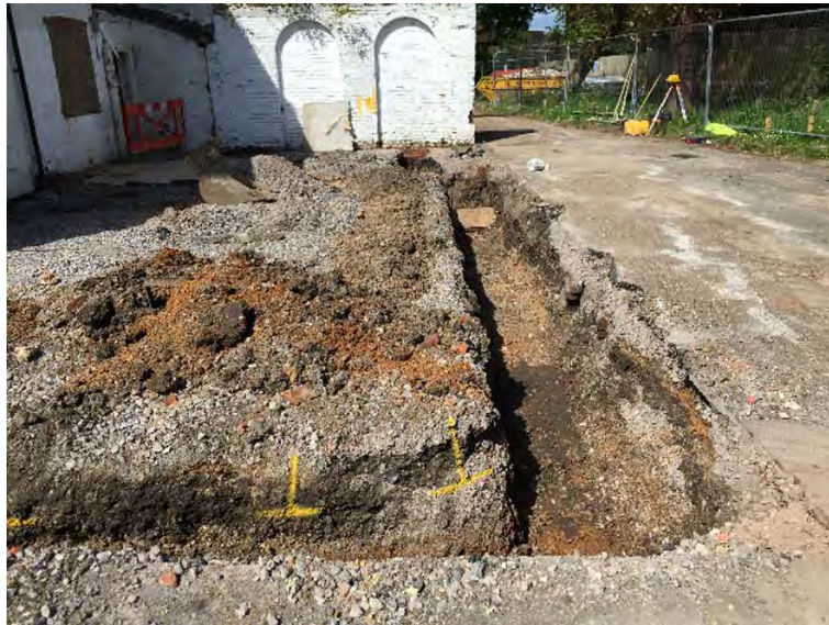
Plate 2. Foundation trenches. West view
