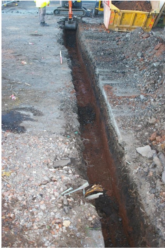
Plate 2. Working shot of service trench
