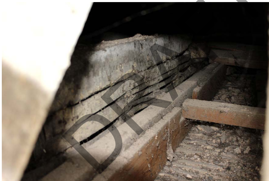
Plate **: internal lath partition visible below collar beam in western room.
