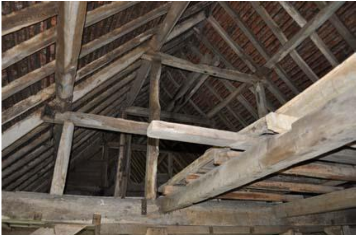
Plate 15: Queen and princess struts on Bin Floor
