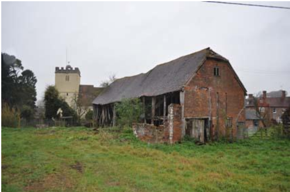
Plate 1: The west and south façades
