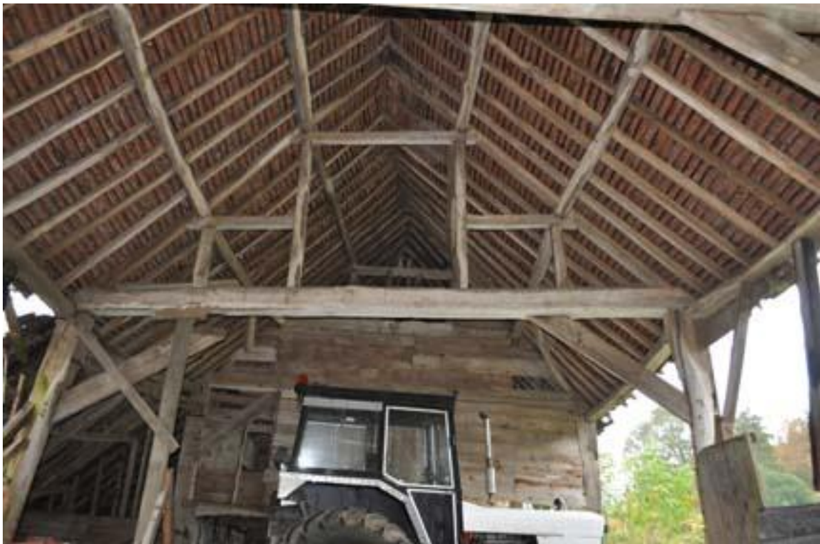
Plate 7: Interior of barn, north wall of mill
