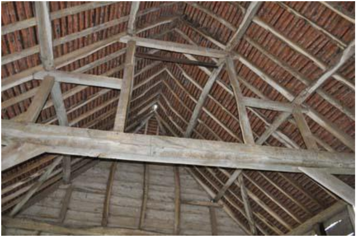
Plate 6: Queen and princess struts, interior barn
