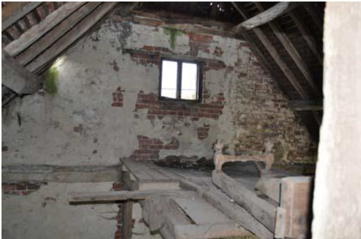
Plate 17: Window in south wall of Bin Floor
