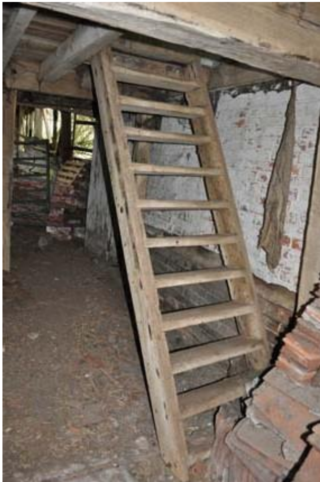
Plate 12: Ladder stairs, Spout Floor
