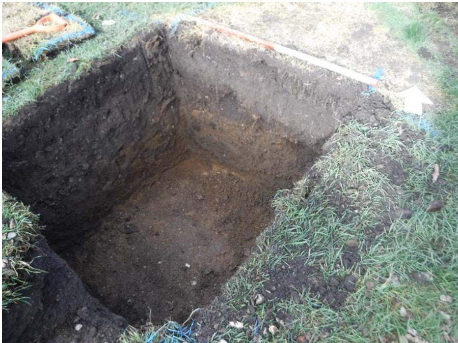
Plate 2: Section 3: Soakaway 3, looking north.
