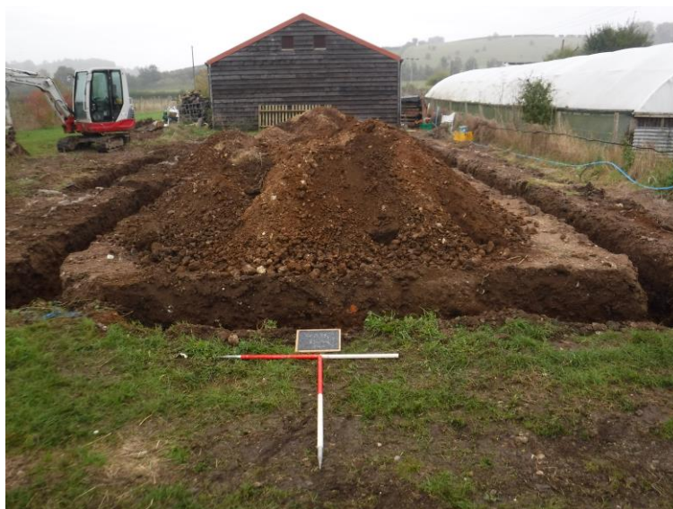
Plate 1: Location of footings, looking northeast
