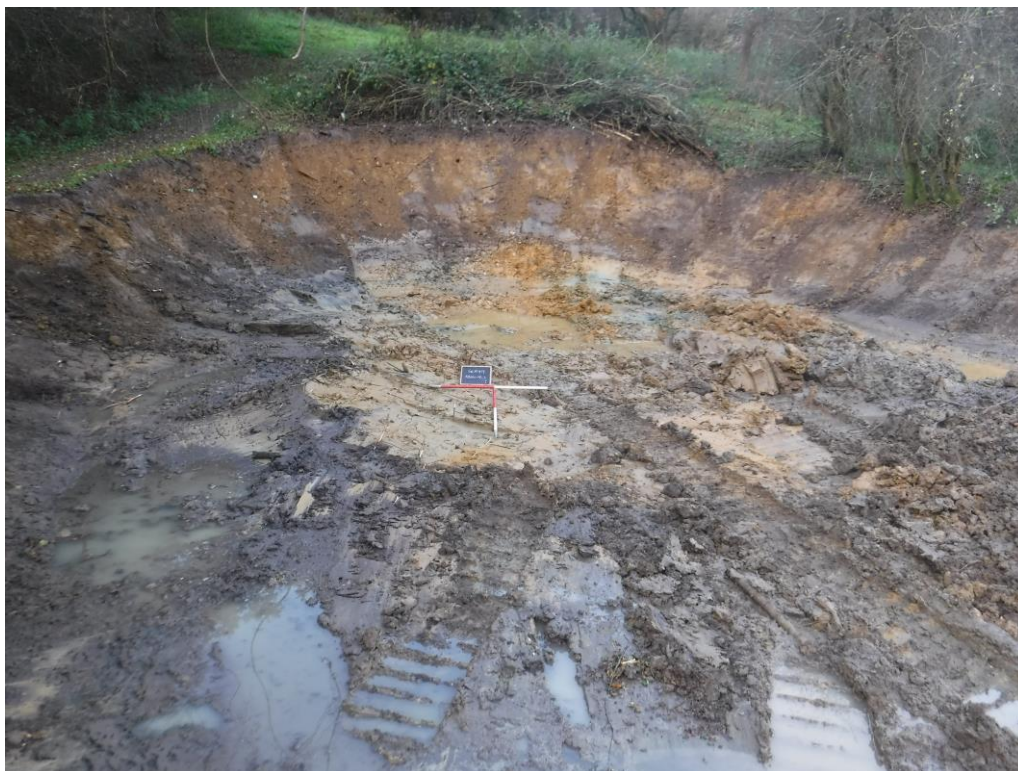
Plate 4. The Completed Groundworks of Pond 3 (RBNW-MP-3).
