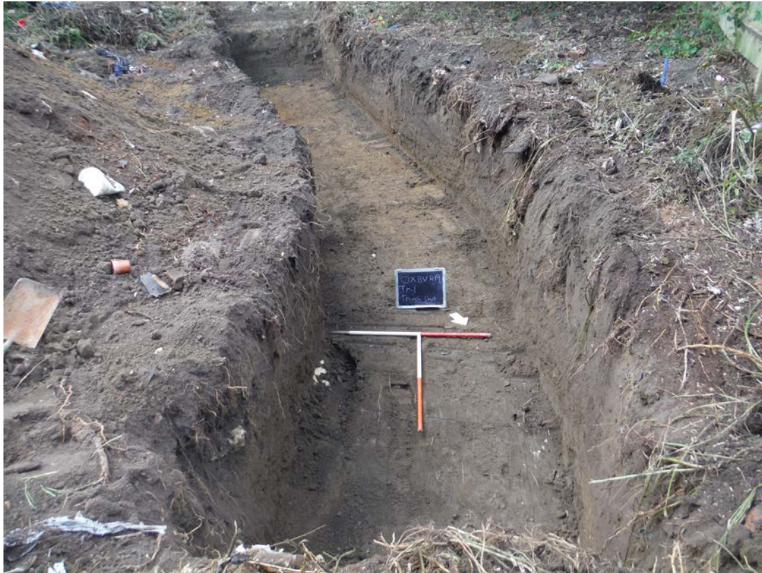
Plate 1: Southwest looking photograph of Trench 1 Pre-excitation
