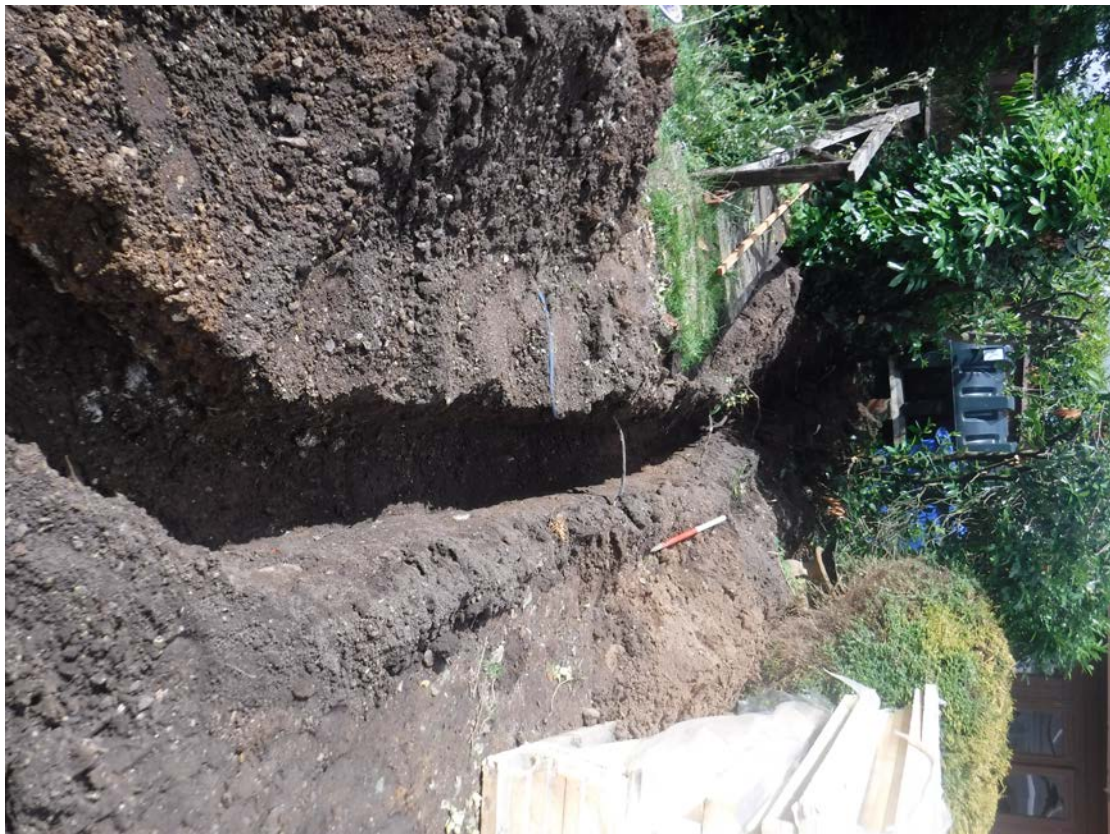
Area 5 – pipe trench
