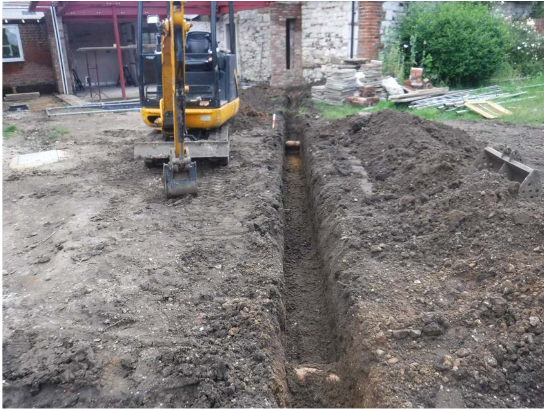
Area 5 – pipe trench
