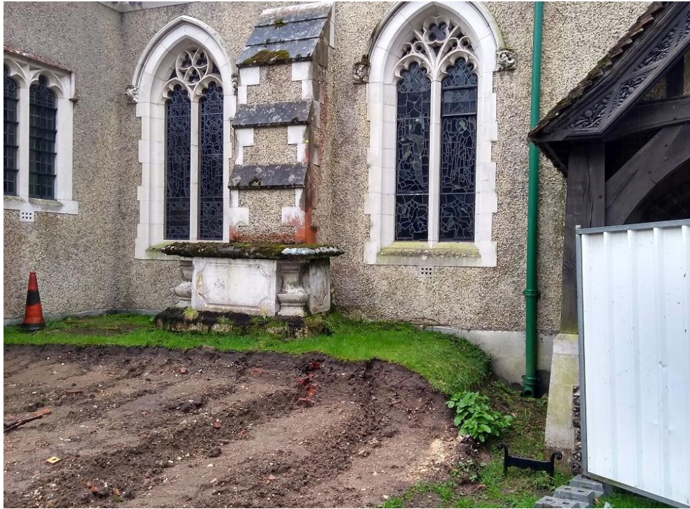
Plate 1. External view of the North Aisle, St. Mary's Church, Wargrave. Flint masonry uncovered during excavation for the reburial of the human remains. Extending at a perpendicular angle to the North Aisle and corresponding to the archway on the internal side of the wall, it is thought to be potentially associated with an earlier architectural layout of the church. View facing south.
