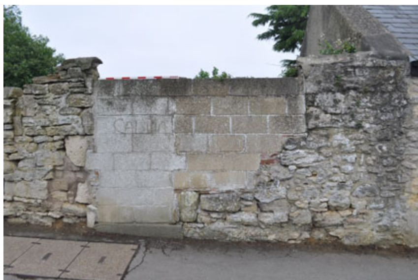
Plate 1: East Face of wall North Part
