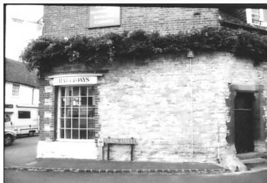
Plate 1: Ground floor clunch construction, first floor of brick. Also shows inserted 20th C. bow window.
