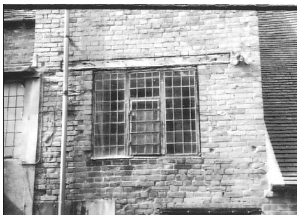
Plate 14: The window on the landing of the 17th century stairway
