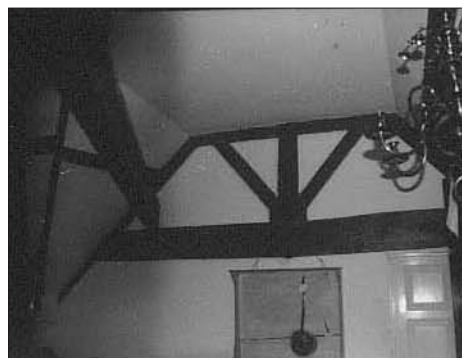
Plate 7: King Post roof construction
