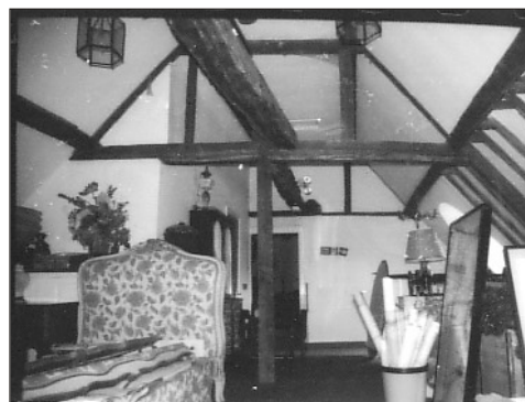
Plate 2: Queen Post roof construction
