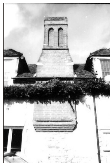
Plate 4: 19th century chimney
