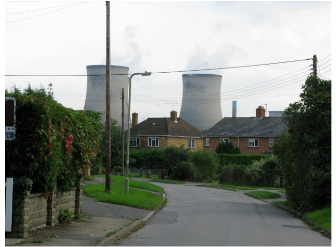
2. View from the historic village of Sutton Courtenay (SU 503 941)
