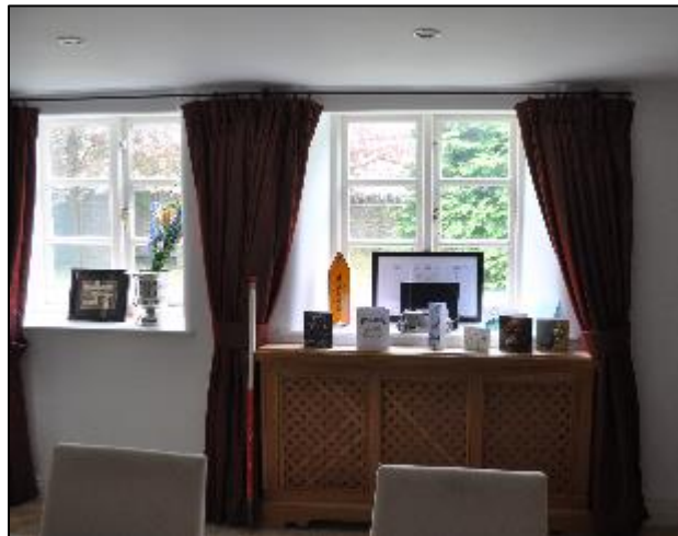
Plate 13 The two double casement windows in Dining Room G3
