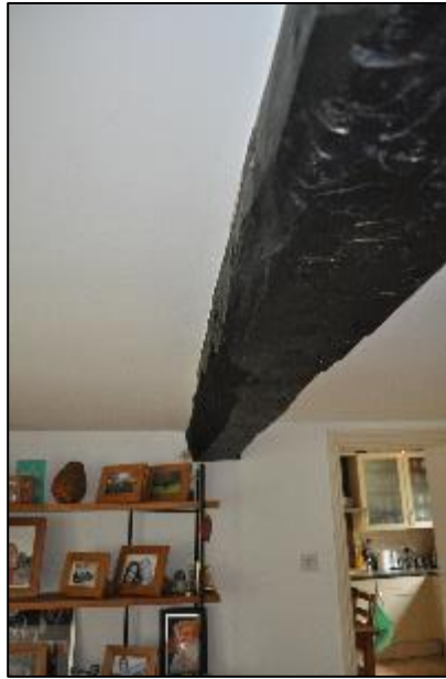
Plate 14 A Close up of the Chamfered dark timber beam in G3 leading towards kitchen G4
