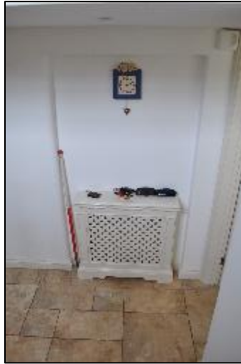
Plate 20 The blocked up hallway entrance that previously led to the main entrance G1 and now contains WC G2. Scale 1m
