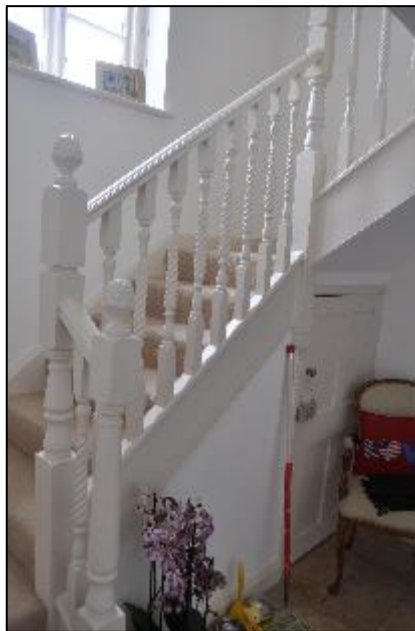
Plate 19 The staircase is an open string, with twisted and turned bannisters with pineapple finials, all painted white. Note the cupboard under the stairs. Scale 1m
