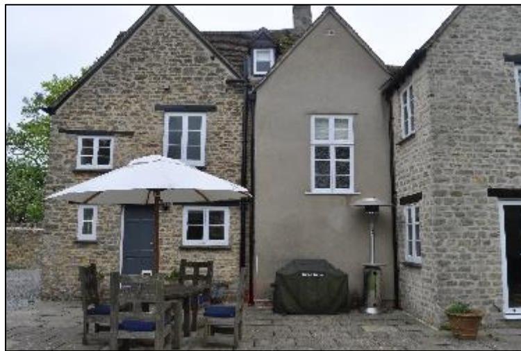
Plate 7: Face Wings 1 & 2 and part of Face Wing 3 of the Northern Elevation
