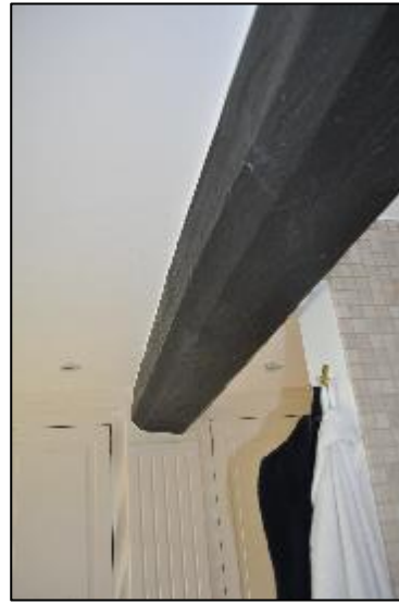
Plate 24 (Left): The modern stain glass window in the double casement window frame in bathroom F4. (Right): The chamfered ceiling beam running east-west in bathroom F4.
