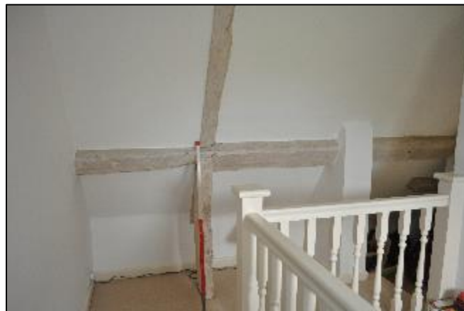
Plate 32: The exposed beams in S1 the southern wall.
