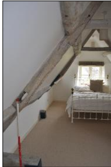
Plate 27 The two sawn-off beams on the ground level of room S2 looking west. Scale 1m
