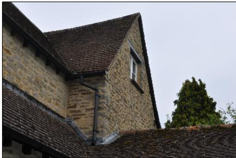
Plate 9 The corner of the Eastern Elevation and Northern Elevation showing the staggered windows (above) and butt joint link to the Face Wing 1
