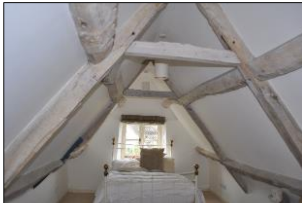
Plate 26 The Roof structure of room S2 looking west
