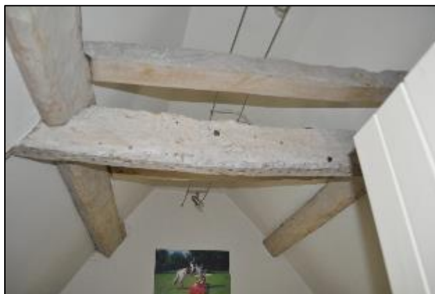
Plate 38: The exposed ceiling beams in S3
