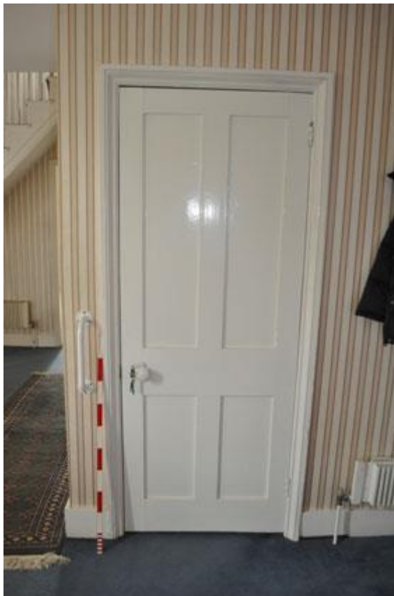
Plate 12: Door in west wall of landing
