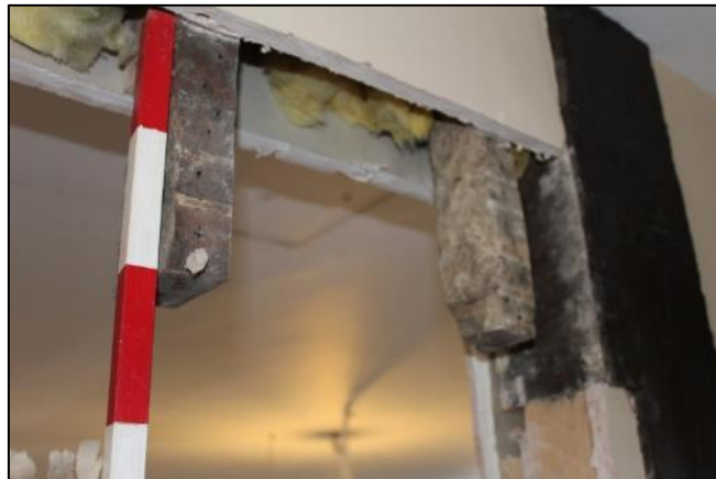
Plate 12: The 17 th C rafters in situ
