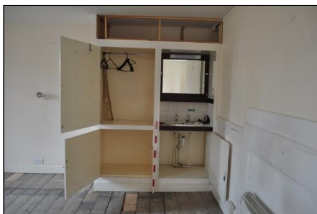
Plate 5: The Cupboard now removed where new door inserted during Watching Brief
