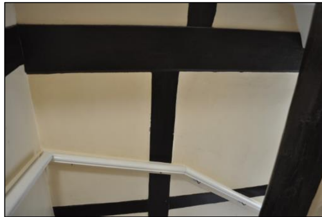
Plate 3: Detail of the timber framing in the stairwell
