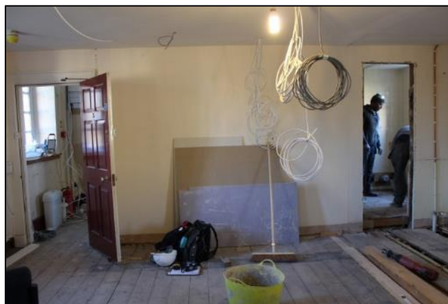
Plate 15: The completed doorway (right)
