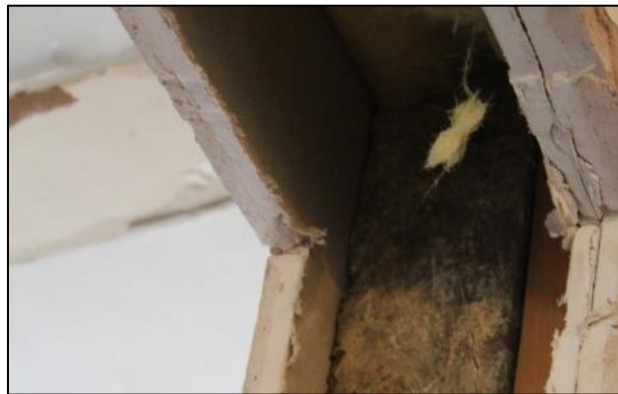
Plate 14: The historic timbers within the thick wall cavity
