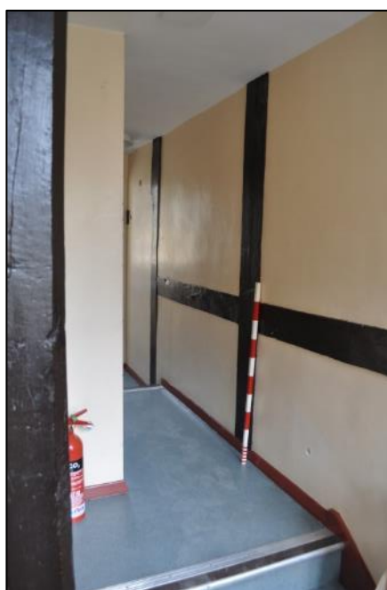
Plate 8: Existing Elevation B showing the historic wooden framing in the corridor towards the bathroom
