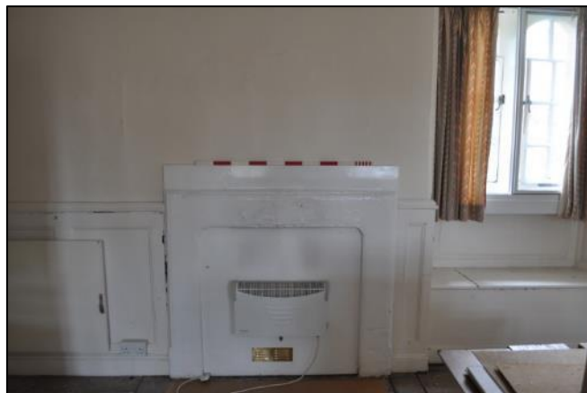
Plate 6: The blocked up fireplace and lancet window
