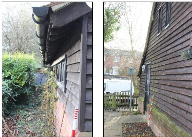
Plate 8: Left: The South-East Elevation and (right) the North-East Elevation
