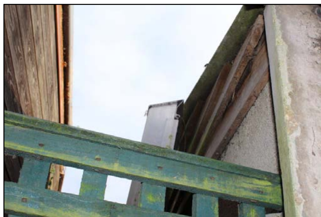
Plate 13: Wood plank panels underneath the roof of shed on north-western gable
