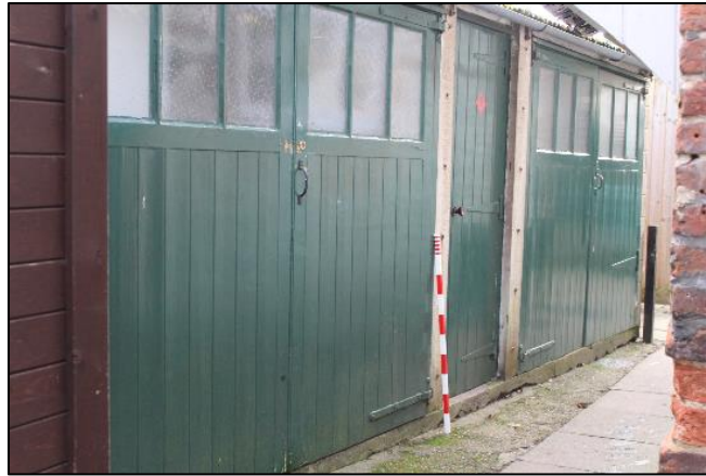
Plate 11: The Sheds South West Elevation
