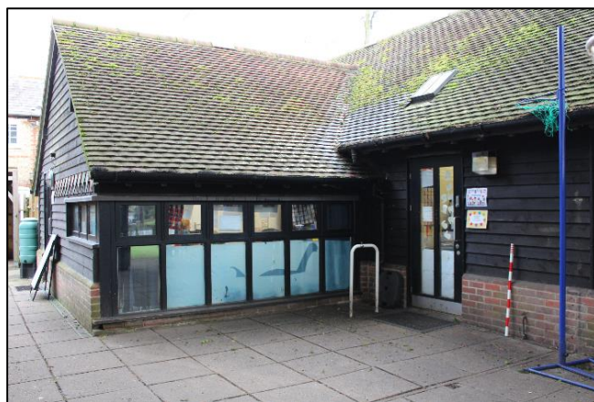
Plate 6: The External Classroom South-West and North-west corner Elevation showing the L-shape
