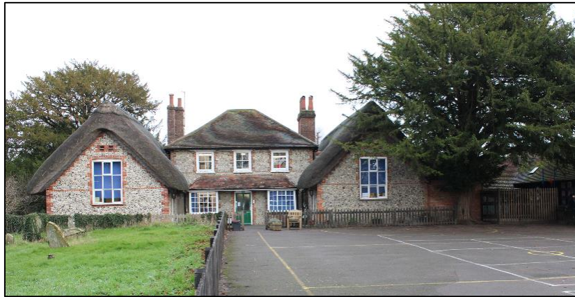
Plate 1: The Main Schoolhouse and two flanking classrooms to north and south
