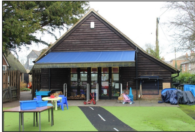
Plate 7: The External classroom South West Elevation showing the outshoot to the south-east
