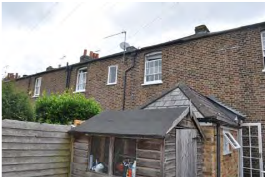
Plate 5: Rear of properties to the west
