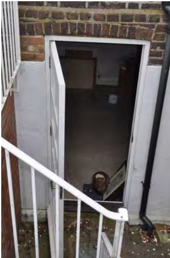
Plate 2: Door into rear light-well
