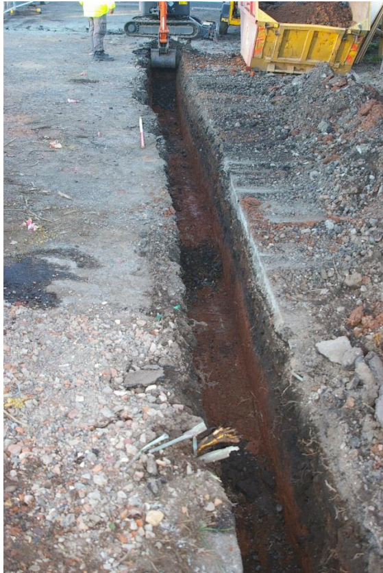
Plate 2. Working shot of service trench
