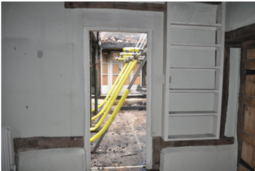
Plate 15: Timbers in west wall of G4
