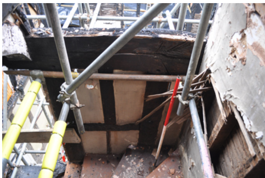
Plate 37: Timbers within the stairwell
