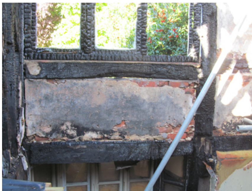
Plate 36: Infilled panel
