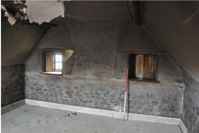
Plate 39: North wall of A1
