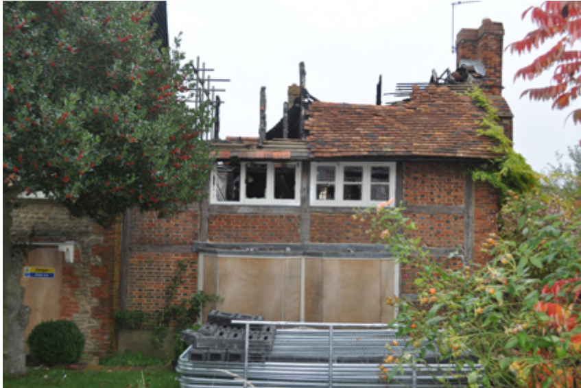
Plate 2: South side of west elevation
