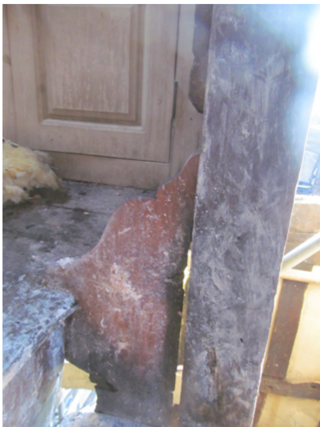
Plate 38: Backplate on stairs
