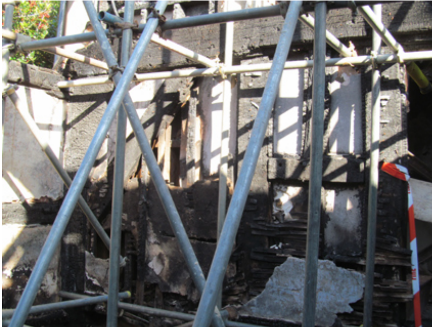
Plate 34: North wall of F3
