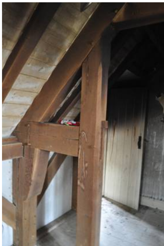
Plate 32: Timbers in F2 creating walkway
