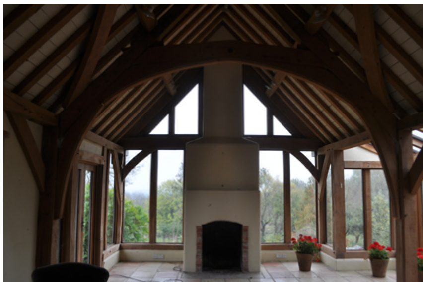
Plate 12: Roof space and fireplace of conservatory (G1)
