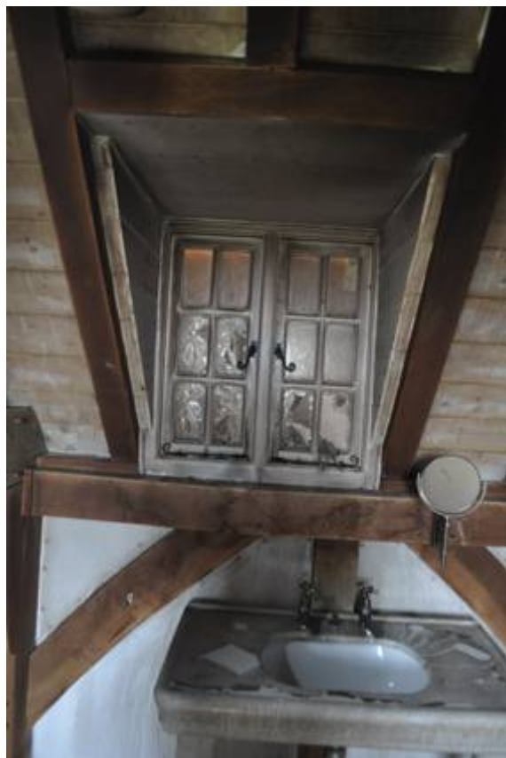
Plate 33: Window in south wall and timbers
