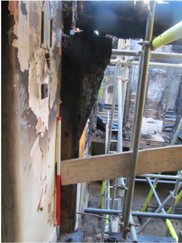
Plate 29: East side of south wall of landing
