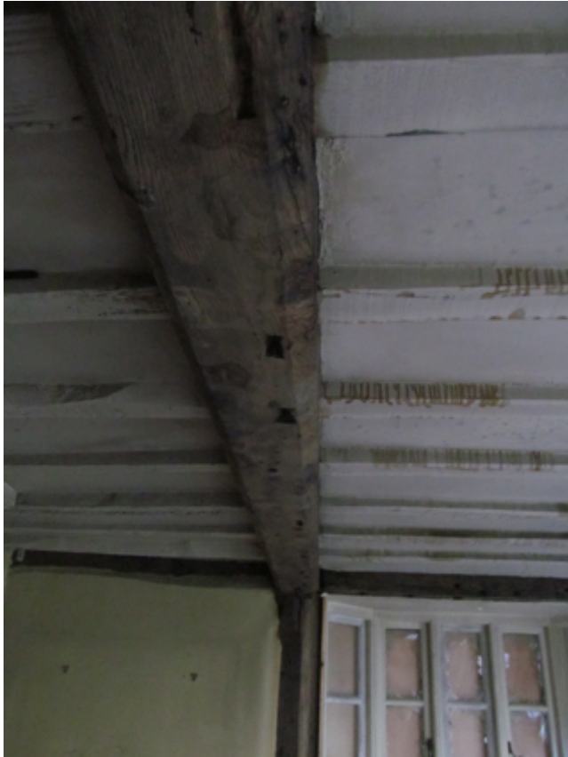
Plate 21: South transverse beam in G5
