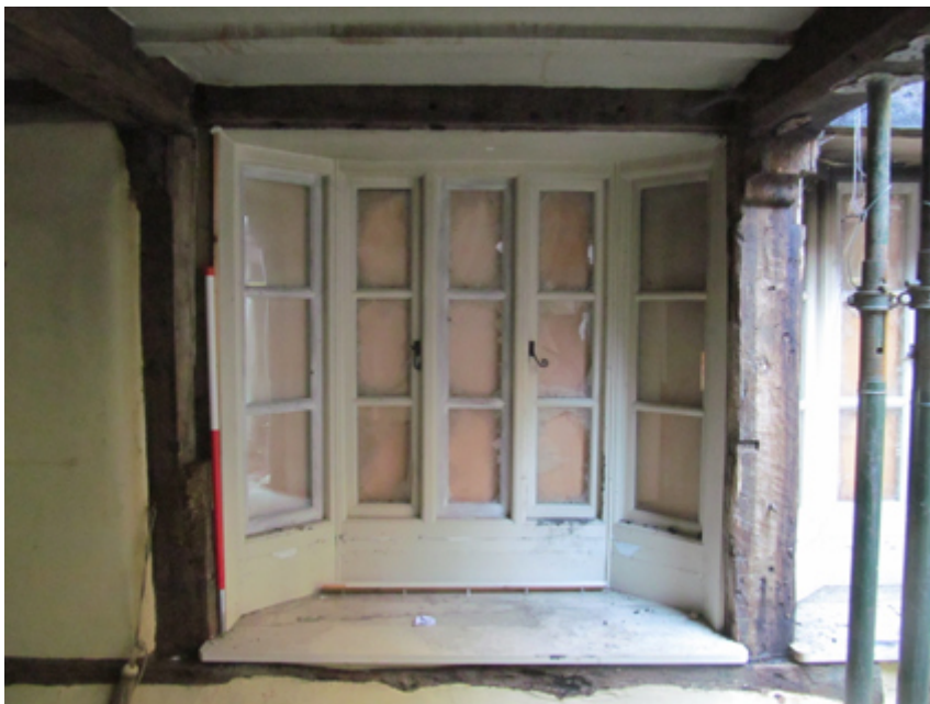
Plate 19: South bay window with cut
