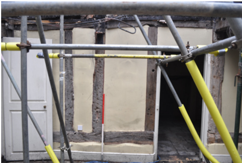
Plate 17: Timbers in east wall of G5
