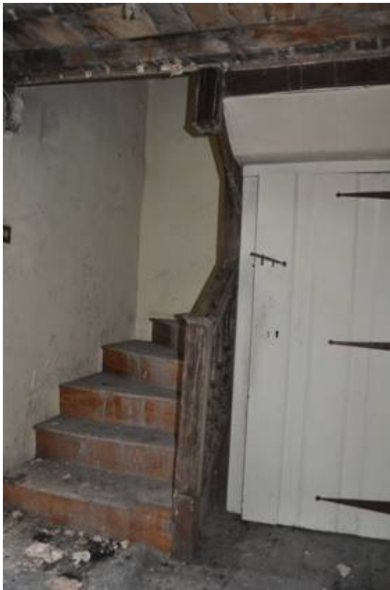
Plate 27: Stairwell at ground floor
