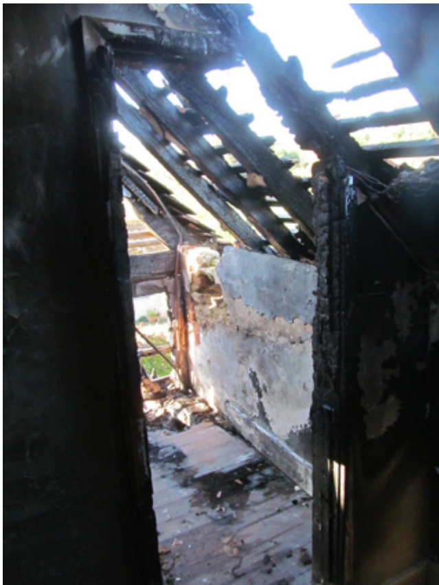
Plate 40: West wall of A2
