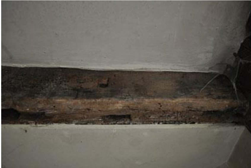
Plate 49: Mortise joints for stud posts
