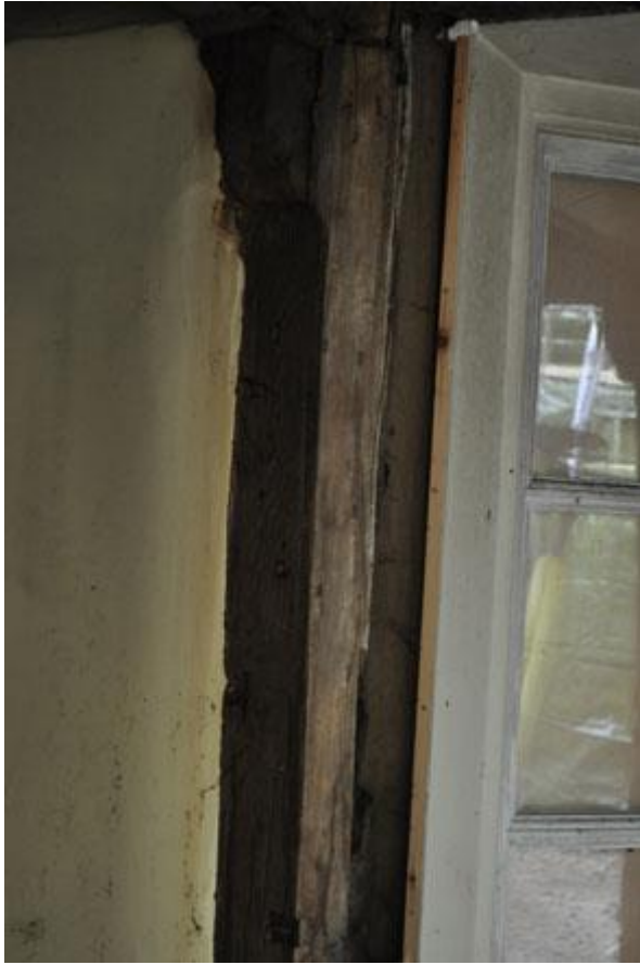
Plate 47: Chamfered post on side of original window
