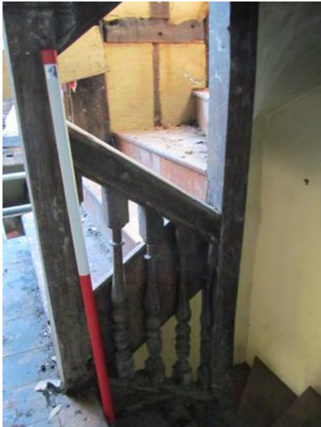
Plate 52: Newel post and turned balusters, with timber frame window behind
