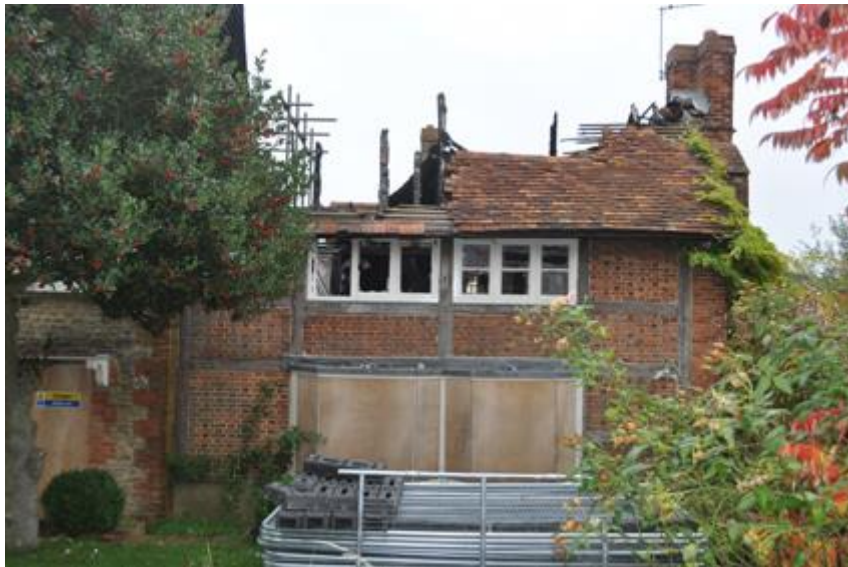
Plate 42: South part of west elevation
