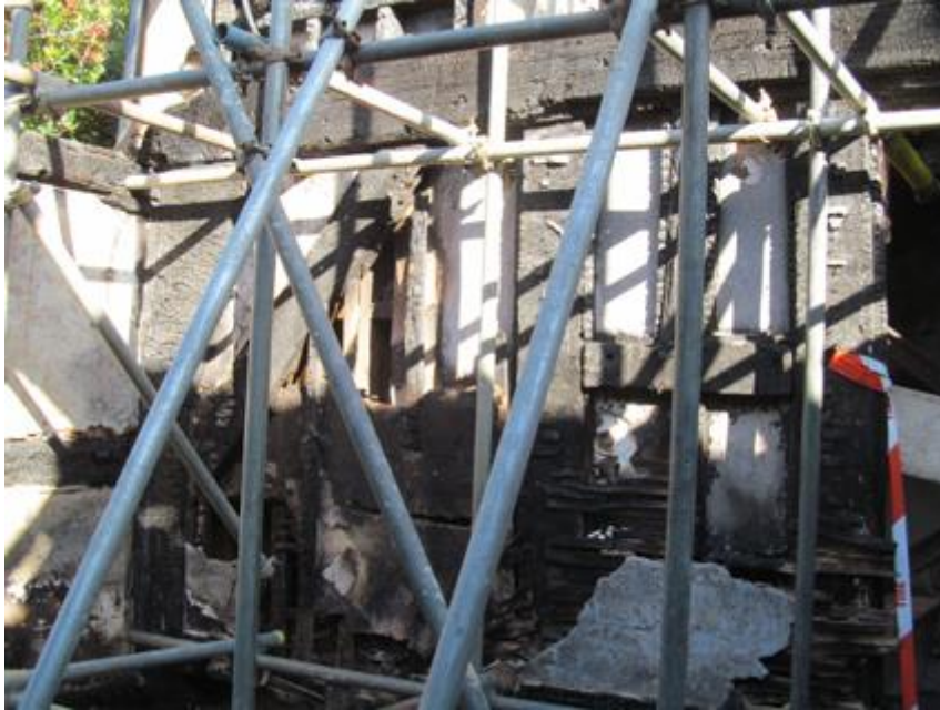
Plate 54: North wall of room F3
