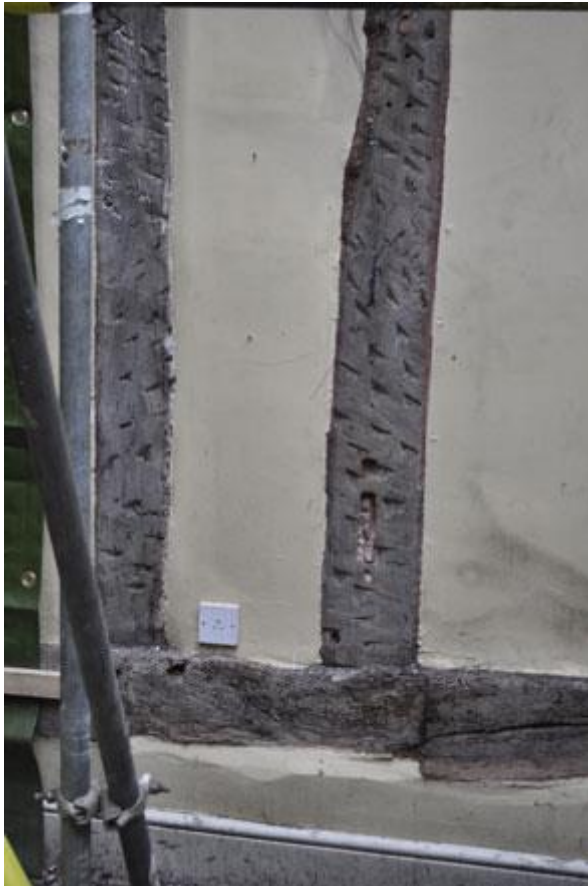
Plate 45: Mortise joint in post
