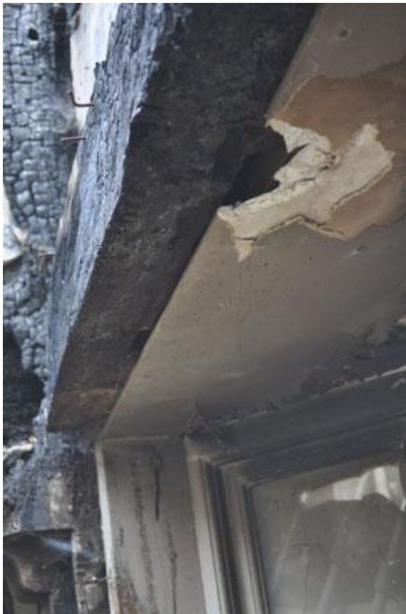
Plate 50: Mortise joints in underside of horizontal beam above north bay window
