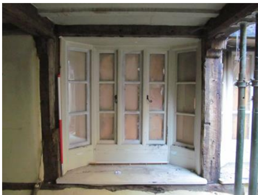
Plate 46: South bay window with cut
