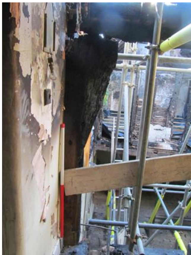
Plate 53: East side of south wall of landing
