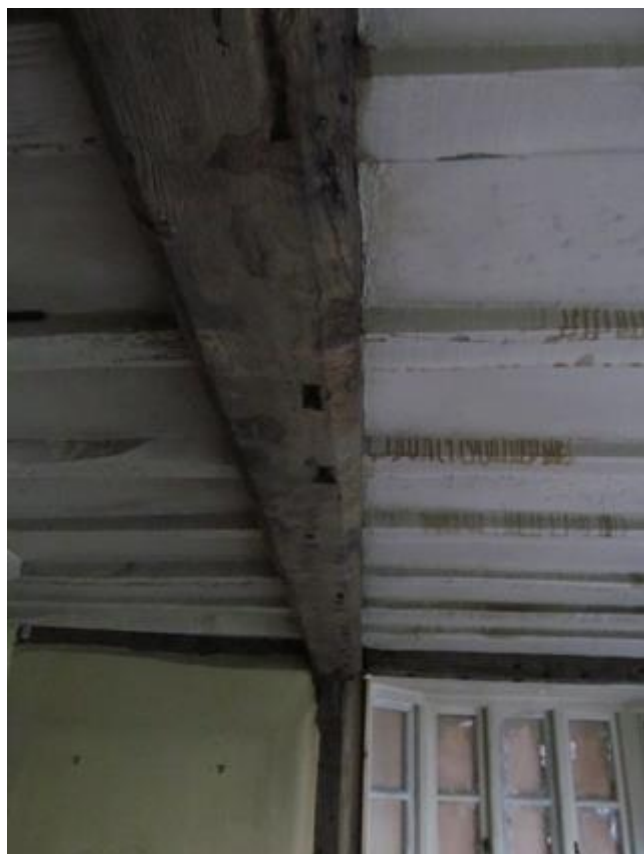
Plate 51: South transverse beam in G5
