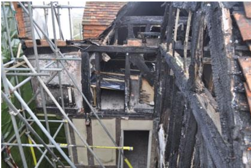
Plate 55: East wall of room F3
