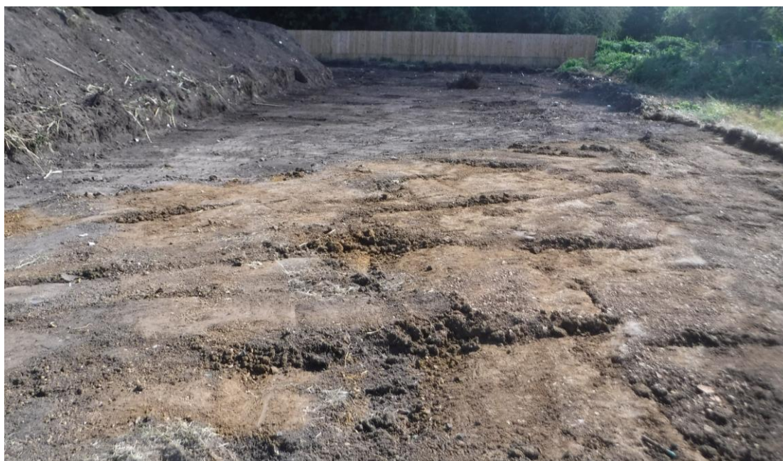
Plate 1: Working shot of dumping pit [04], facing east
