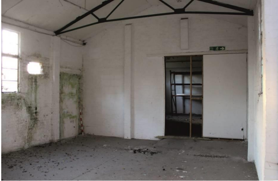
Plate 17: Room B2, north western wall showing truncated buttress. Looking west.
