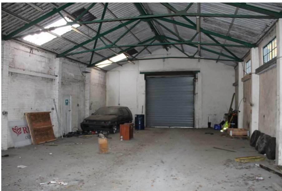
Plate 10: Building A, northern end. Looking north west.
