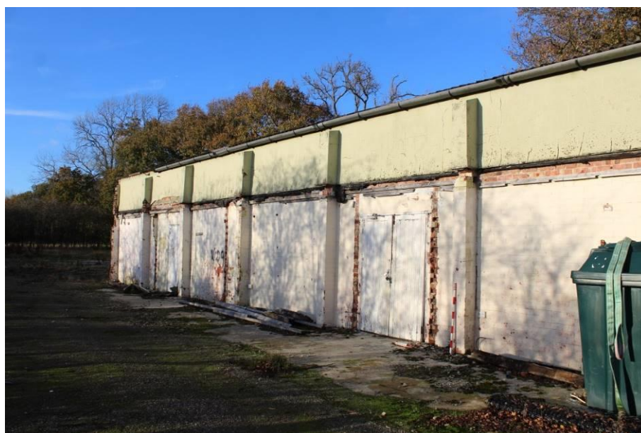
Plate 4: South west elevation, building A. Looking north
