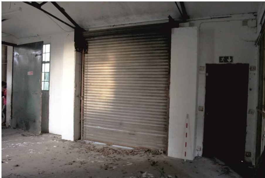
Plate 14: Room B1, north eastern wall. Looking north.
