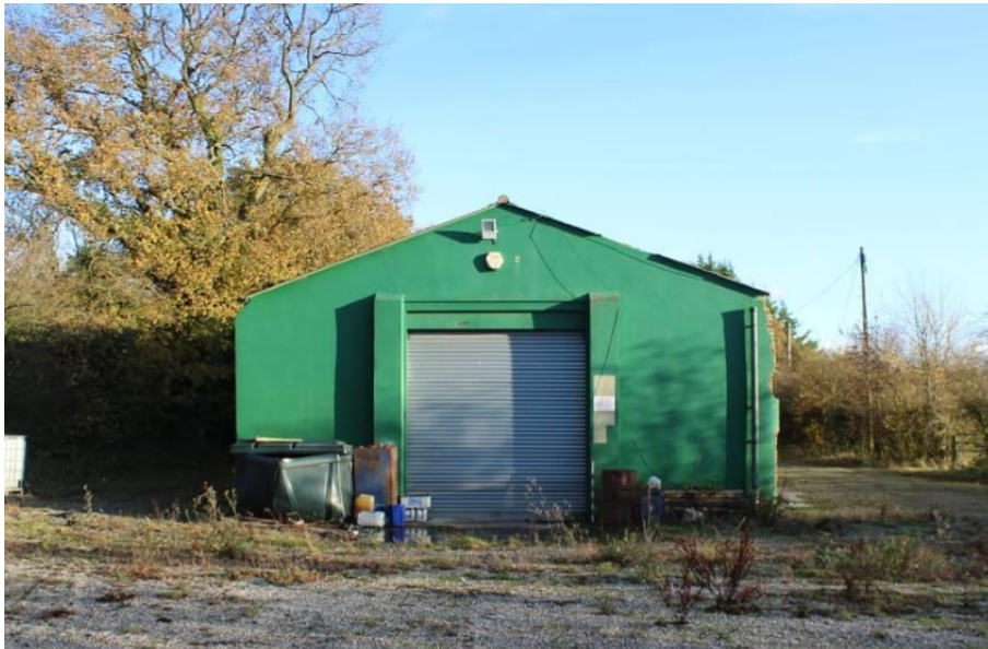
Plate 8: North west elevation, building A. Looking south east
