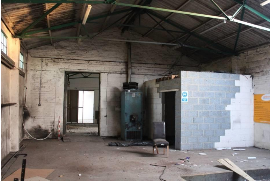
Plate 11: Building A, southern end. Looking south east
