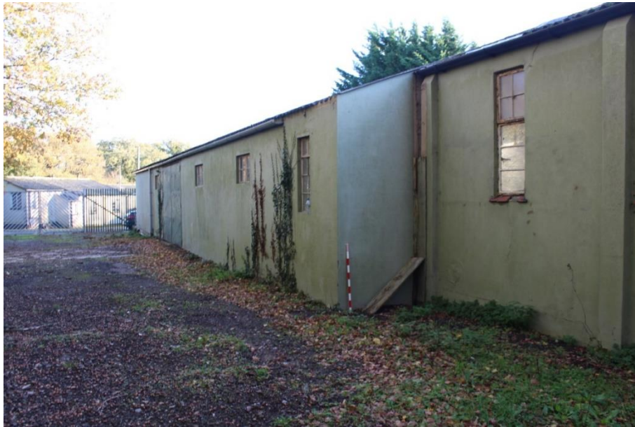
Plate 1: North east elevation, buildings B and C. Looking south.
