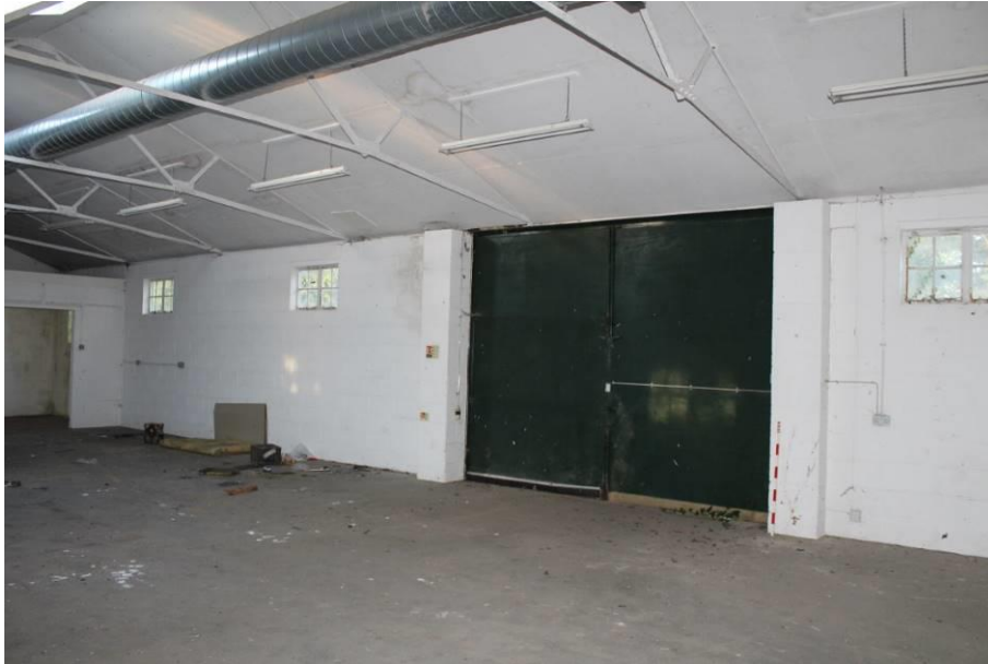
Plate 21: Building C, north eastern wall. Looking north.
