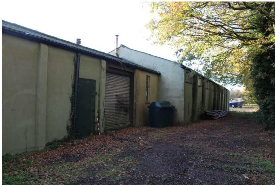
Plate 2: North east elevation, buildings A and B. Looking west.
