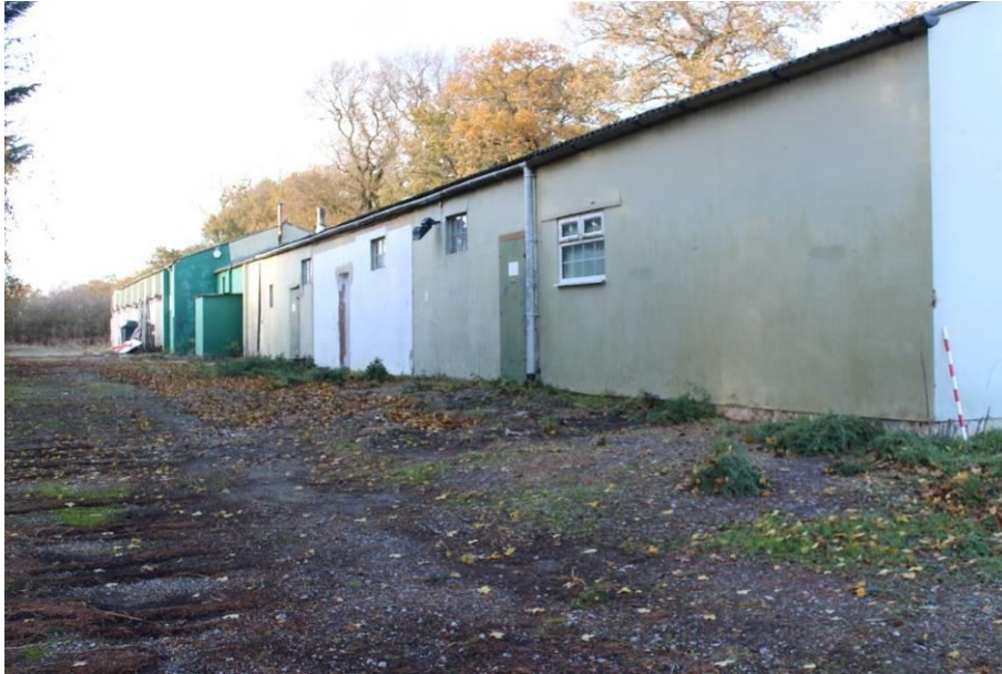
Plate 7: South west elevation, building C. Looking north.
