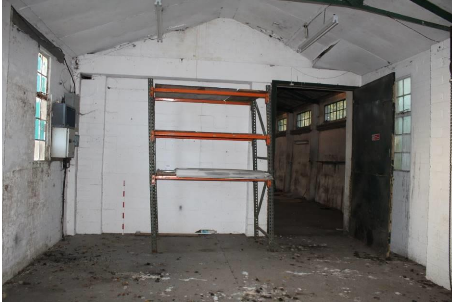
Plate 13: Room B1, north western wall. Looking north west.
