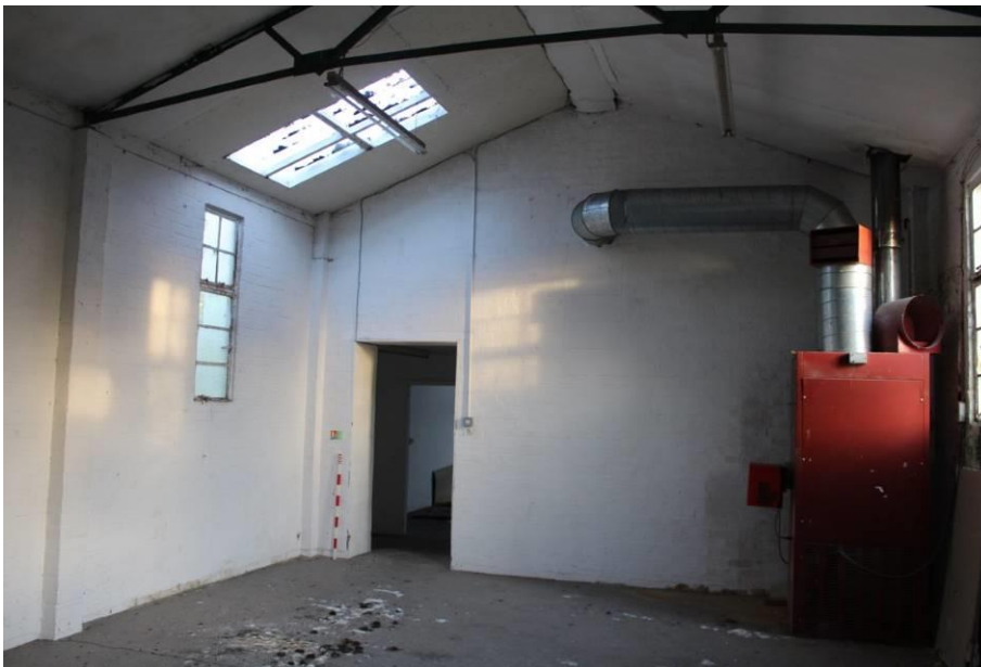
Plate 18: Room B2, north eastern and south western wall. Looking east.
