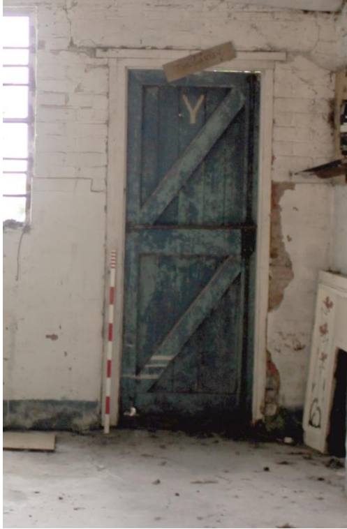
Plate 26: Room G1; northern wall with historic door. Looking north
