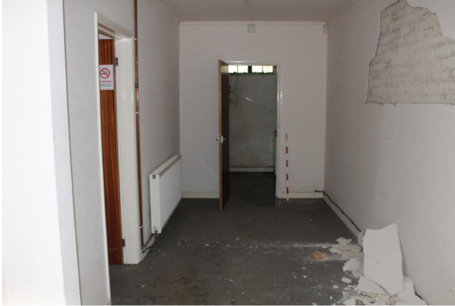
Plate 10: Room A1; showing partitions. Looking north.
