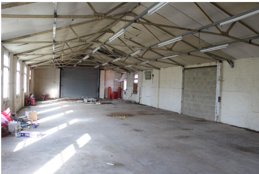
Plate 28: Room H2; showing roof structure and blocked doorway. Looking north.
