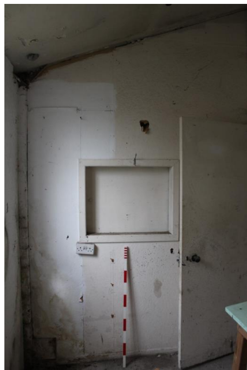
Plate 20: Hatch in room D4; looking north.
