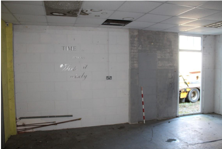
Plate 12: Room B1, northern wall; showing blocked entrances. Looking north
