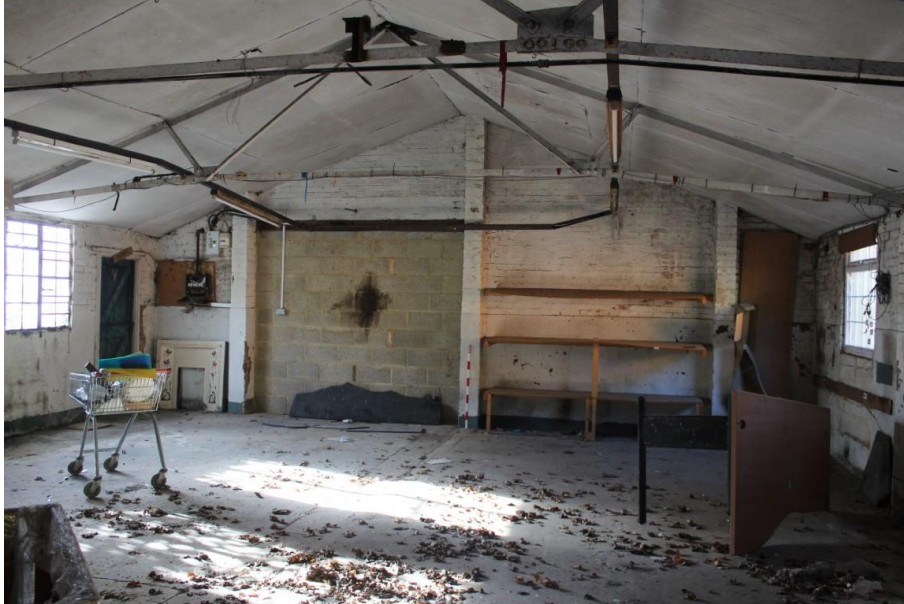
Plate 24: Room G1; west wall and roof structure. Looking west
