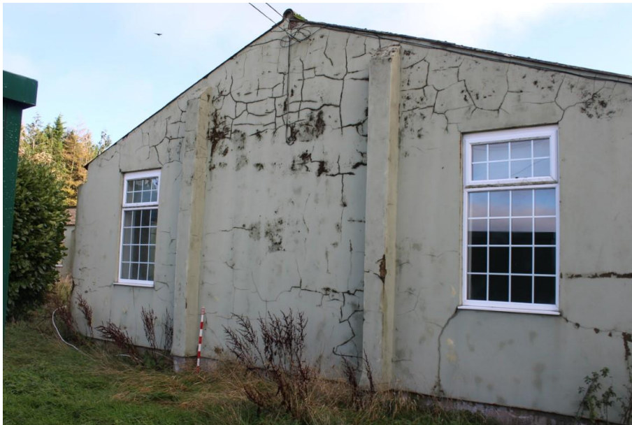
Plate 5: Southern gable end, elevation EE. Looking north east.
