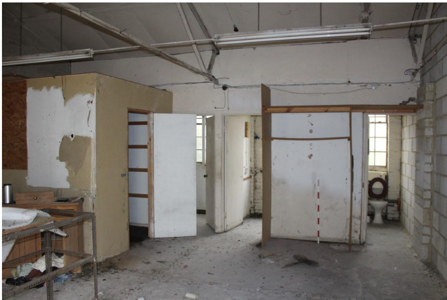
Plate 18: Room D1, partitions D2 to D4. Looking west.
