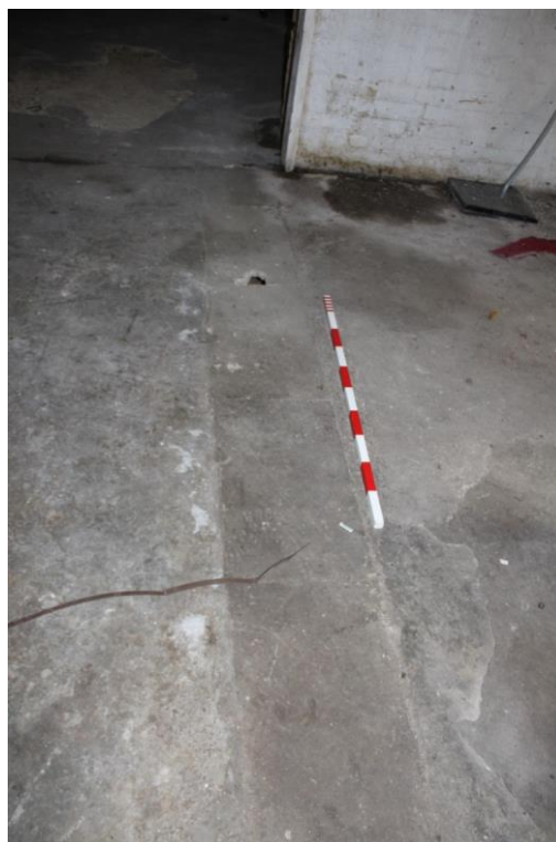
Plate 23: Room E; water pipe trench. Looking east.
