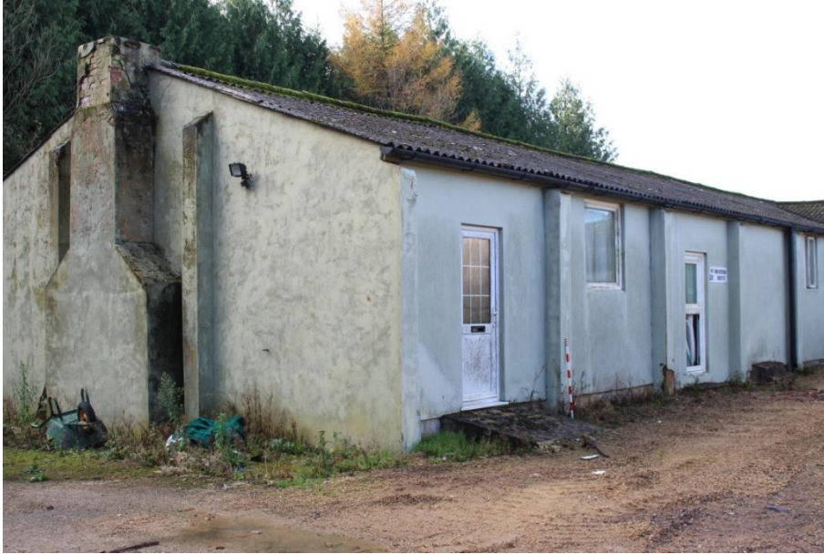
Plate 2: Eastern end of elevation BB and southern end of elevation EE, looking south east.
