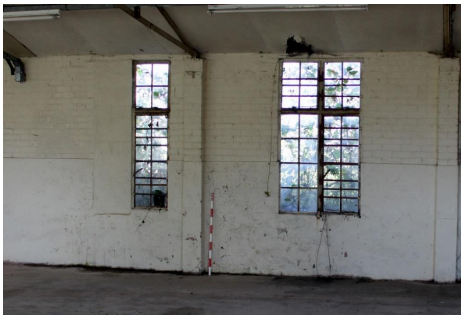
Plate 29: Room H2; eastern wall with historic windows. Looking east
