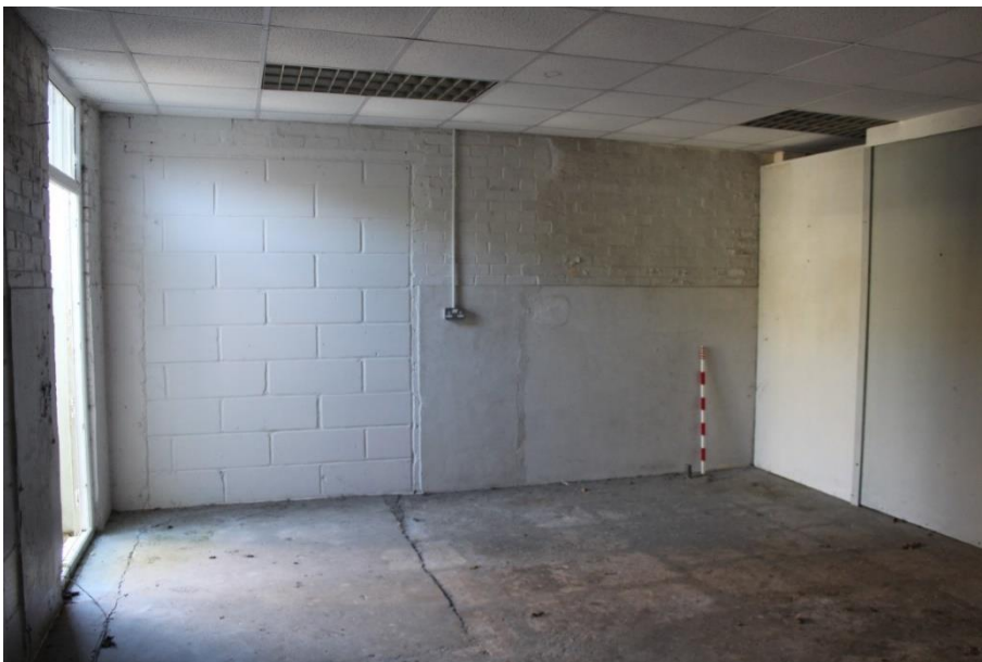
Plate 13: Room B1, eastern wall showing blocked internal doorway. Looking east.
