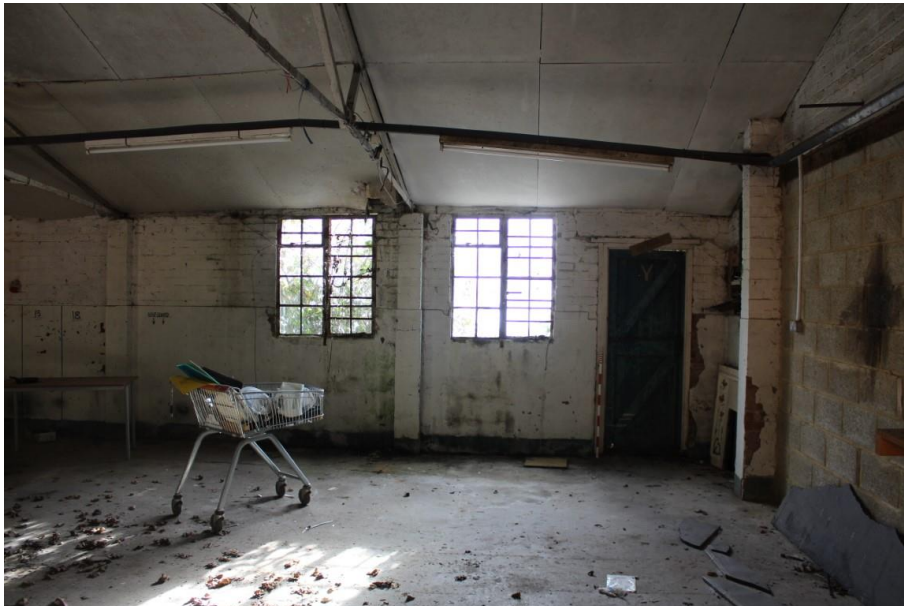
Plate 25: Room G1; southern wall with historic door and windows. Looking south
