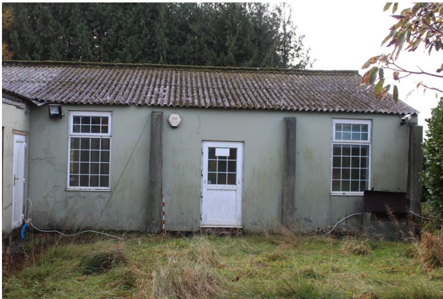
Plate 3: Western end of elevation BB, looking south.
