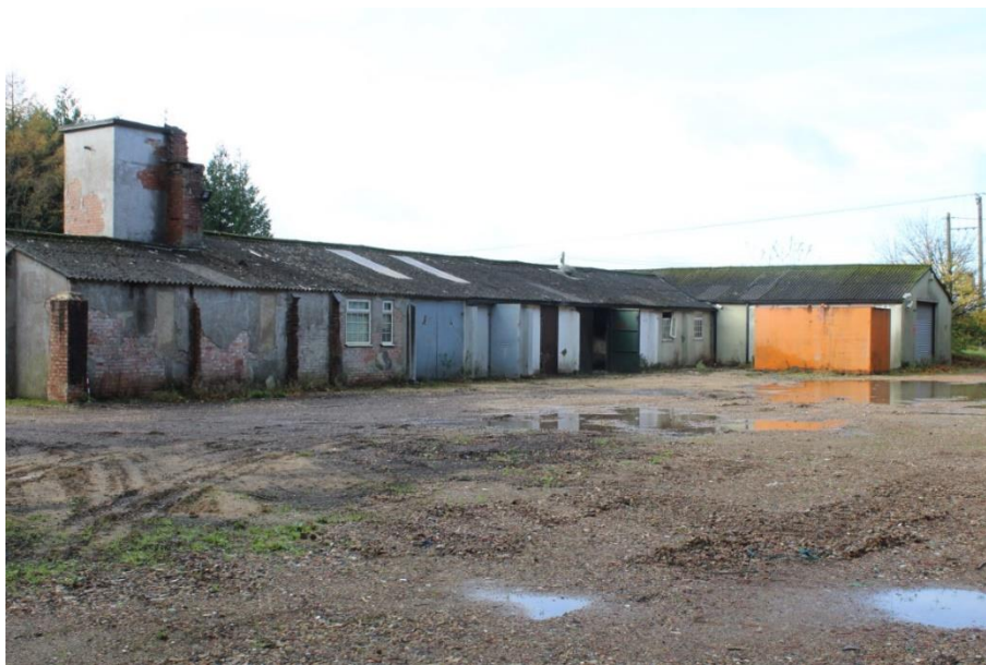
Plate 9: North elevation FF and east elevation EE, looking south west.
