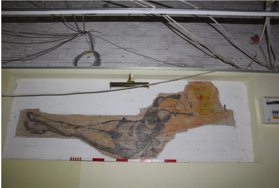
Plate 17: Room C6, western wall; showing extant mural. Looking west.
