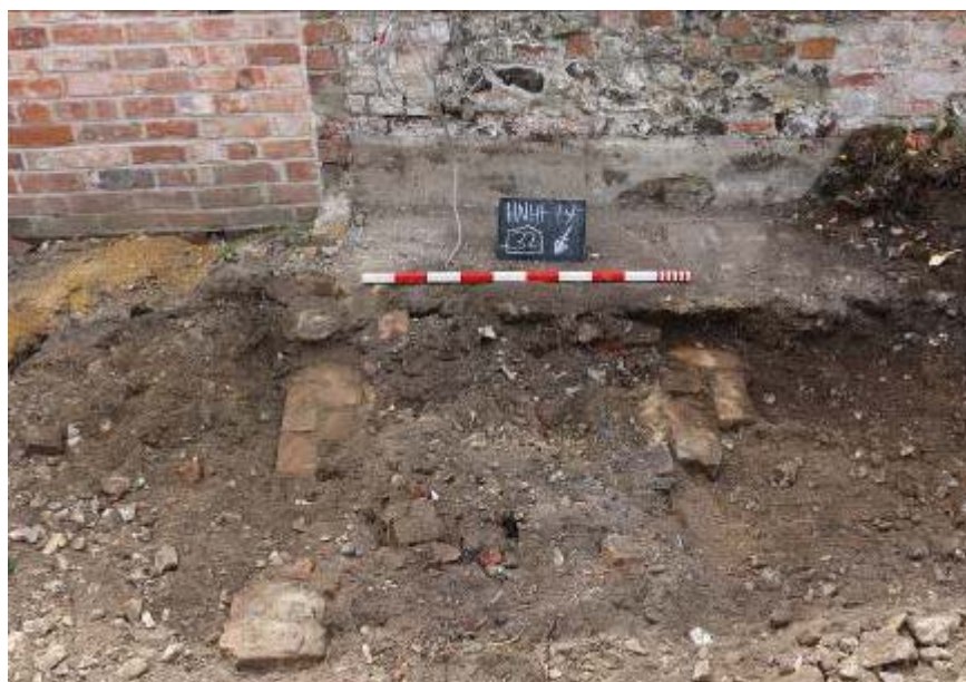
Plate 1: Area 1, foundation footer 32 .
