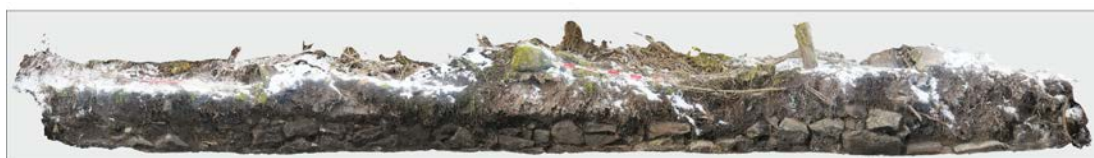
Plate 9: Wall 300 , orthophoto. Looking NW
