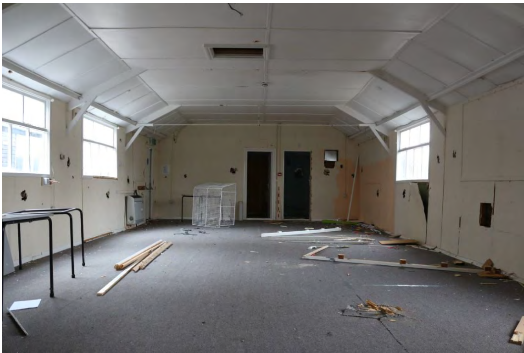
Plate 13: Room 10, showing blocked windows and roof structure. Looking north.
