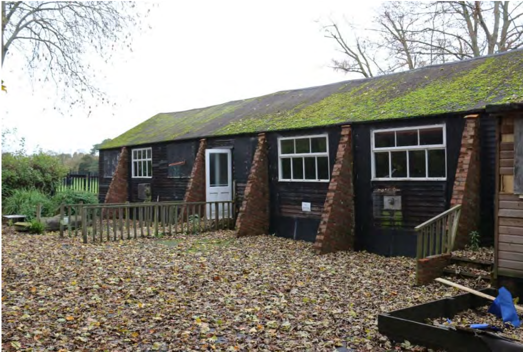
Plate 6: The northern end of the western block, showing buttresses. Looking north east.
