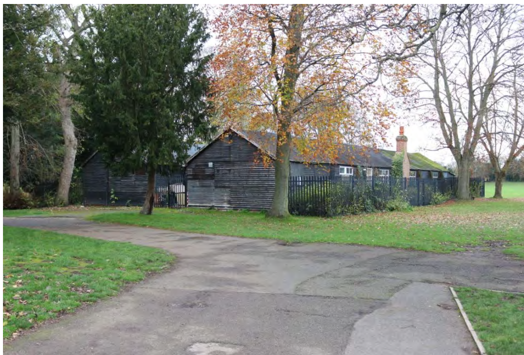
Plate 1: The recreation rooms as viewed from the entrance to The Bullcroft. Looking north east
