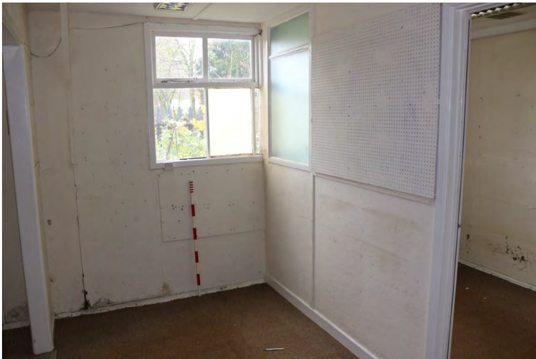
Plate 11: Rooms 6 and 8, showing partition of external window. Looking east.
