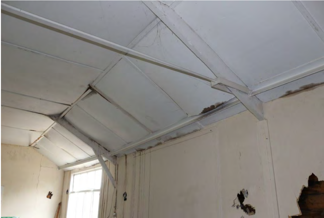
Plate 21: Room 18, showing roof structure and metal tie beam. Looking north east.
