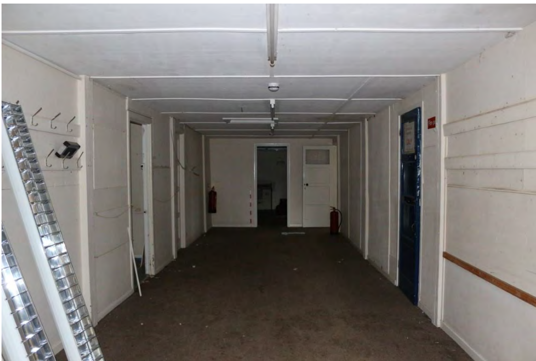
Plate 9: Room 1, central corridor. Looking north.
