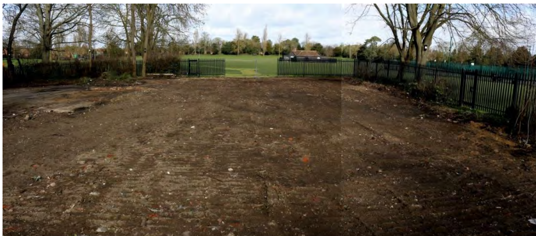
Plate 23: The site, post-demolition. Looking north.
