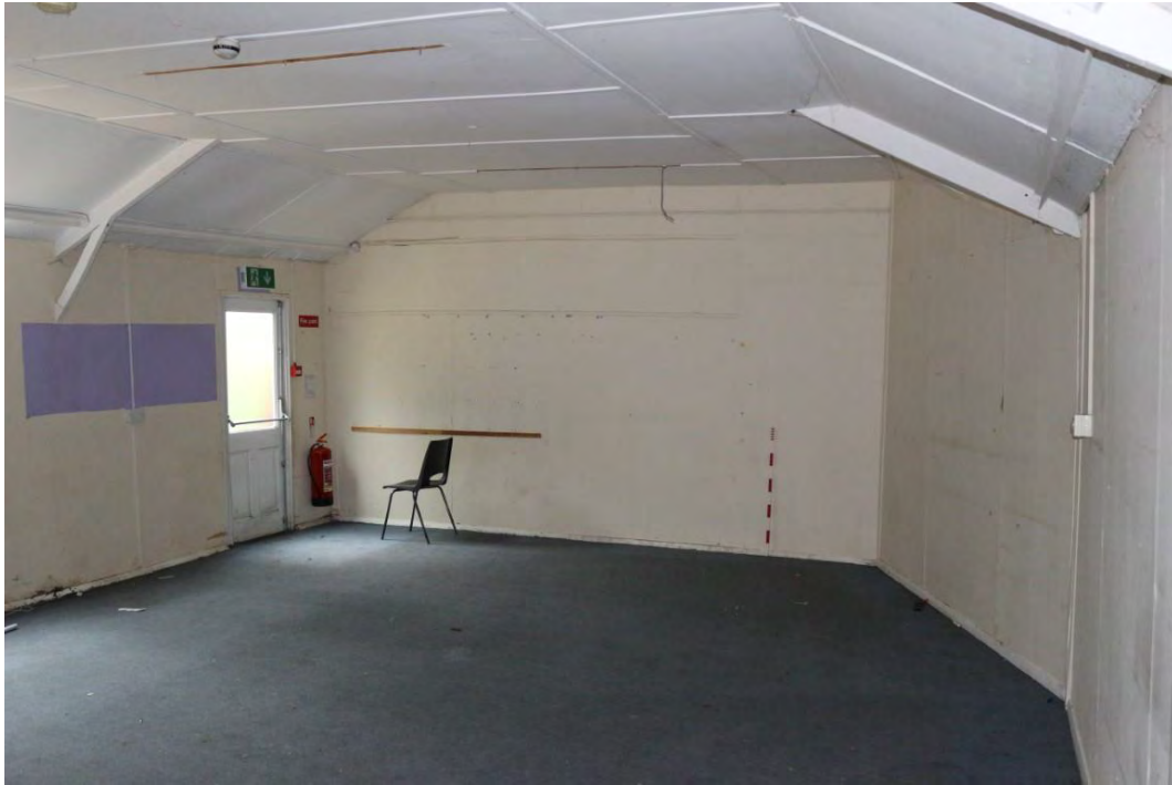
Plate 17: Room 17, showing altered eastern wall. Looking north-north west.
