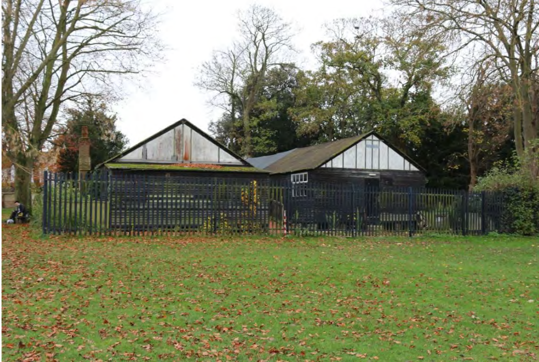
Plate 4: The northern elevation. Looking south-south west
