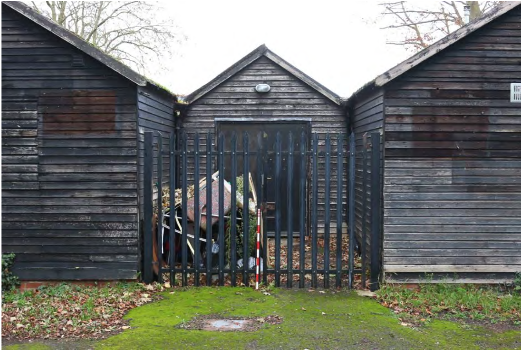
Plate 2: The central entrance into the building. Looking north
