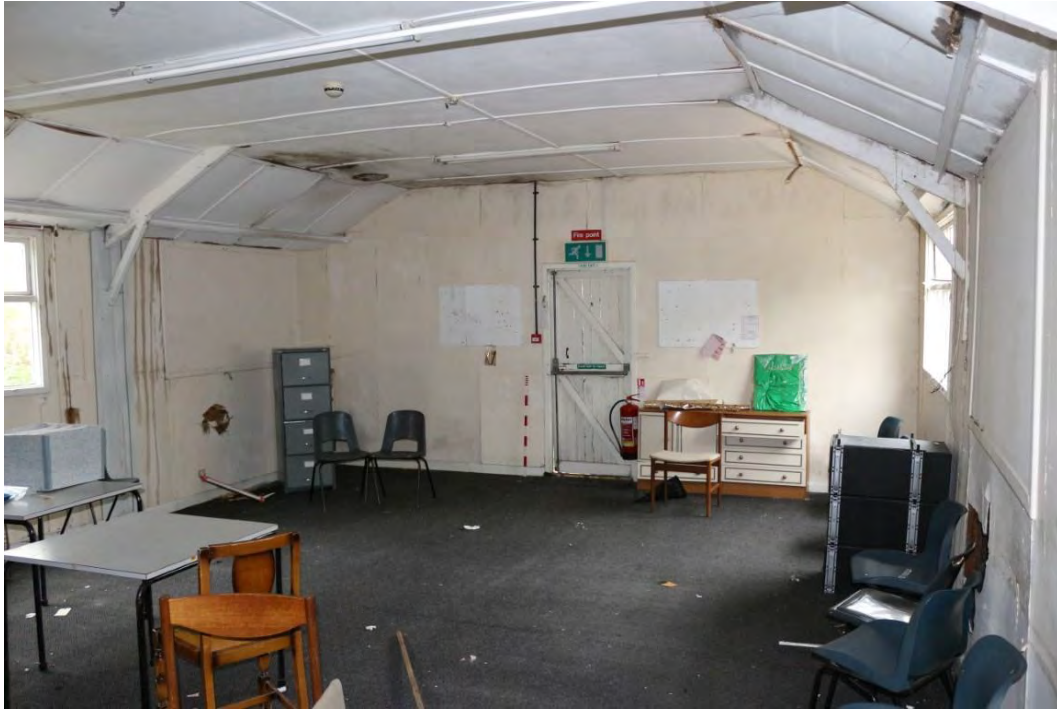
Plate 19: Room 18, showing door and blocked windows. Looking north.
