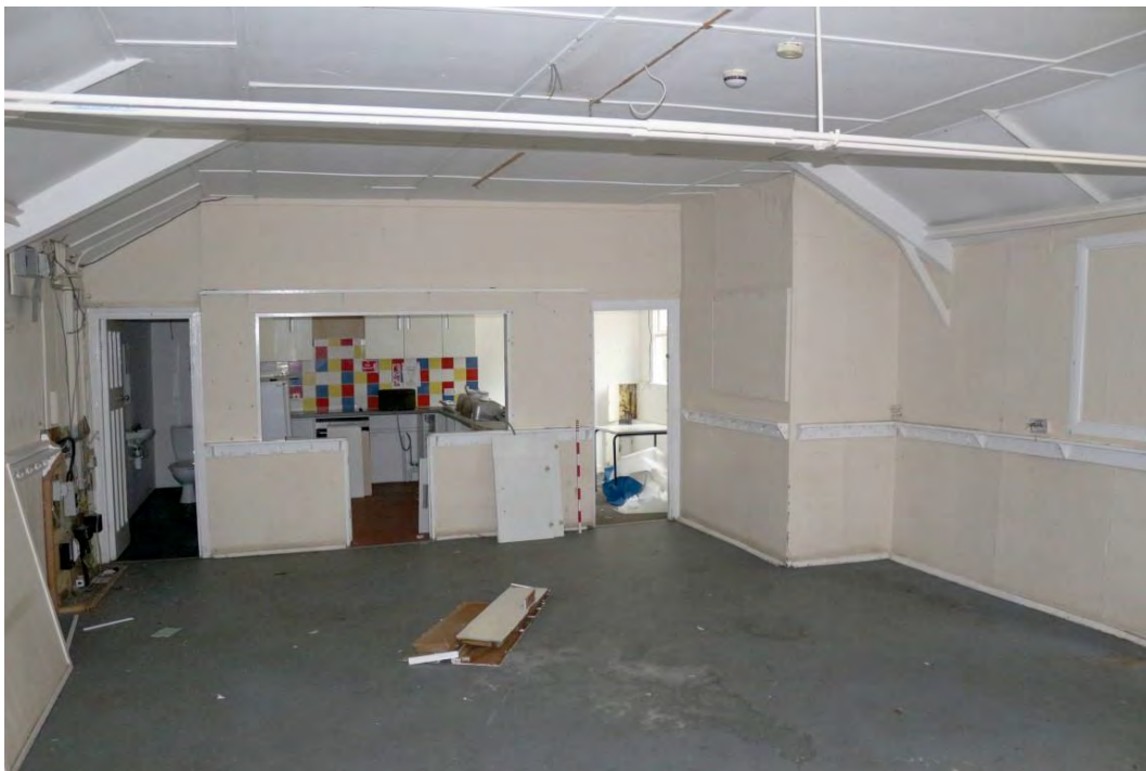
Plate 15: Room 13, showing Toilet 14 and Kitchen 15. Looking south.
