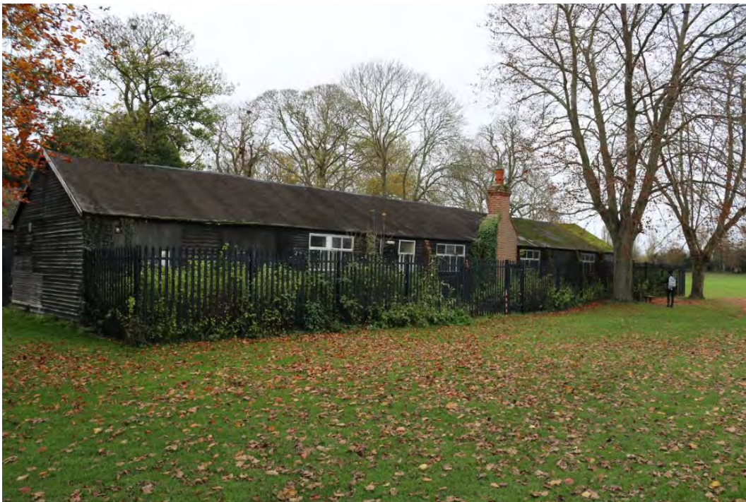
Plate 3: The eastern elevation of the east block. Looking north west
