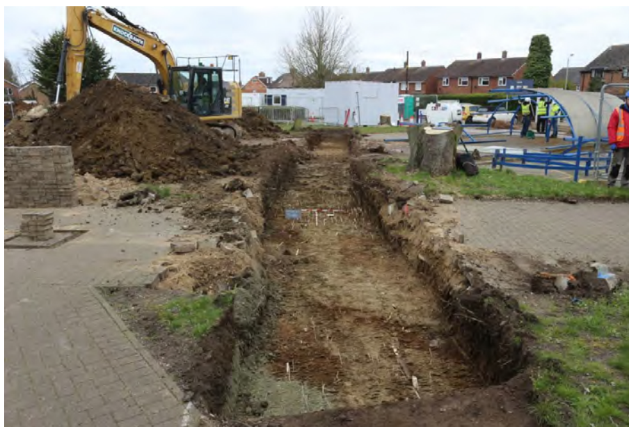
Plate 3: Trench 2; looking south west
