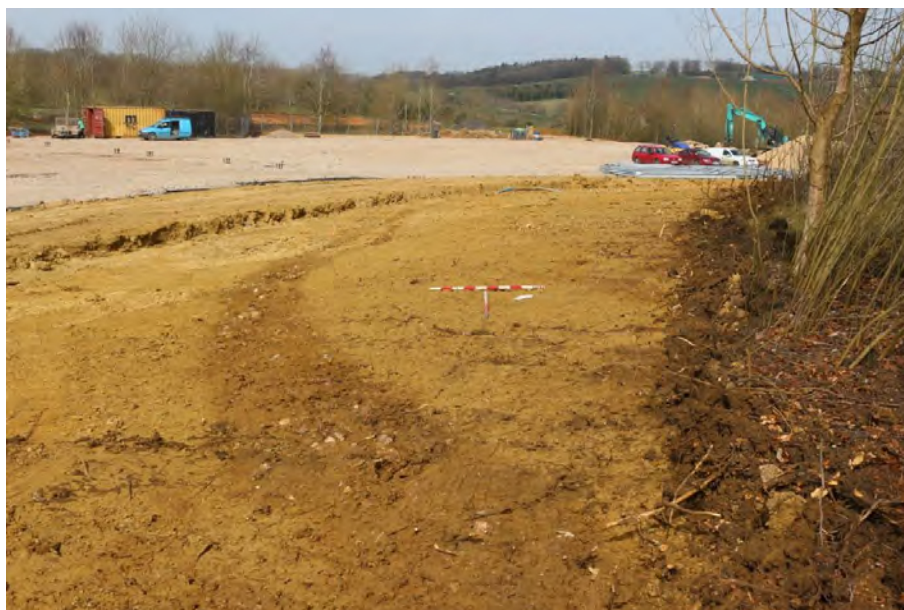
Plate 6: Ditches 22, 24 and 26. Looking north west.
