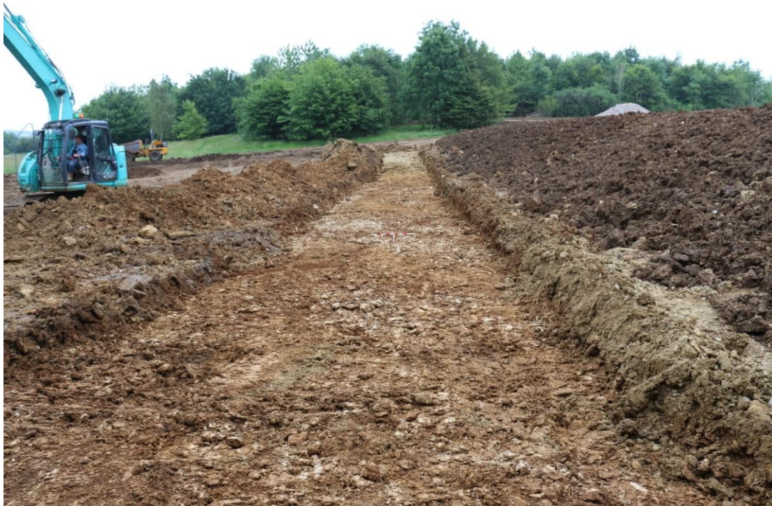
Plate 1: Area of excavation, looking south east
