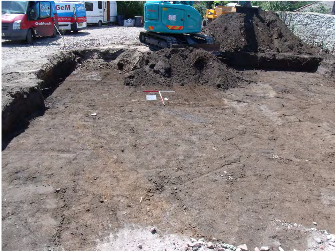
Plate 3: General area of footprint of house. View facing SSW.
