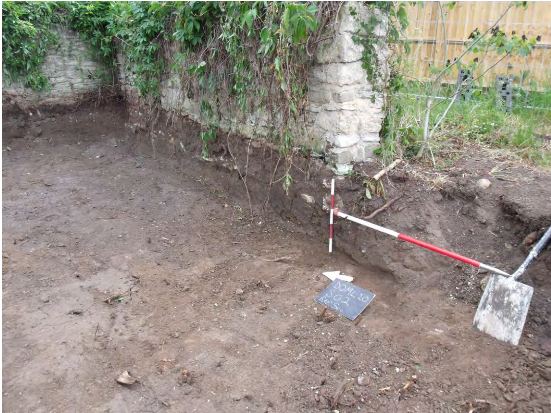
Plate 1: Garage footprint; Section 02, wall 03 , prior to removal. View facing ENE.
