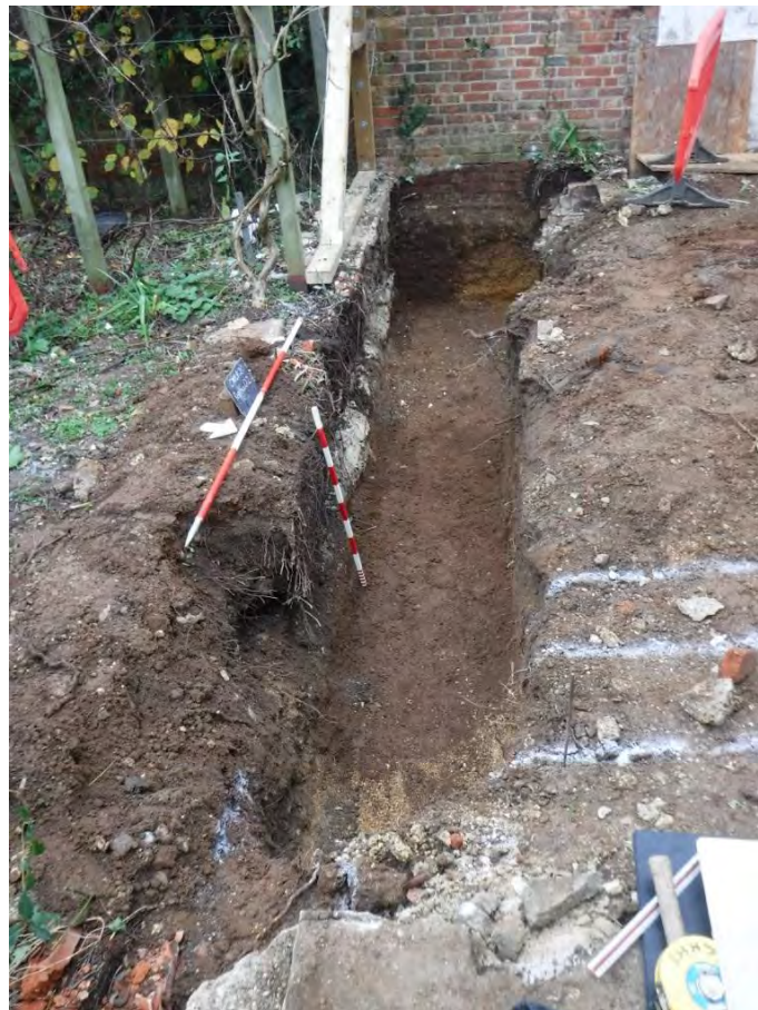
Plate 1: Footings trench. Looking west
