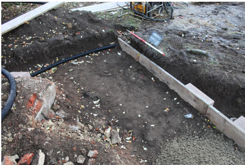
Plate 1: Photograph of reduced area to the rear of the property
