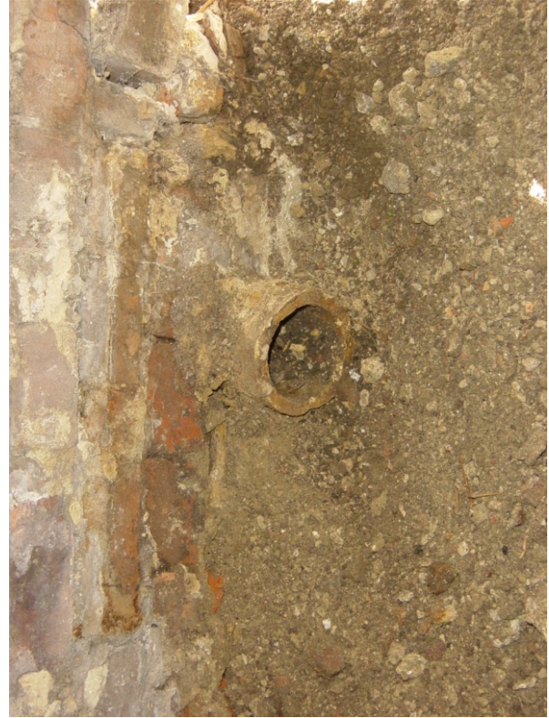
Plate 12. Pipe under flooring in third room
