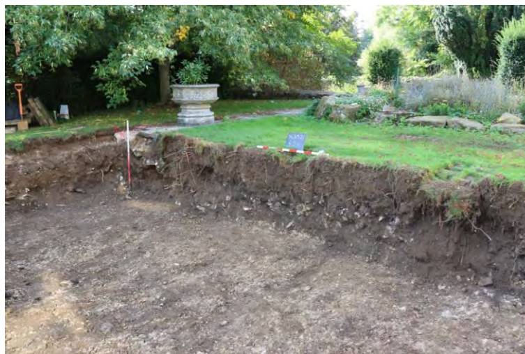
Plate 4: SW end of footprint, showing Section 2 and deposit (02). Looking SSW.
