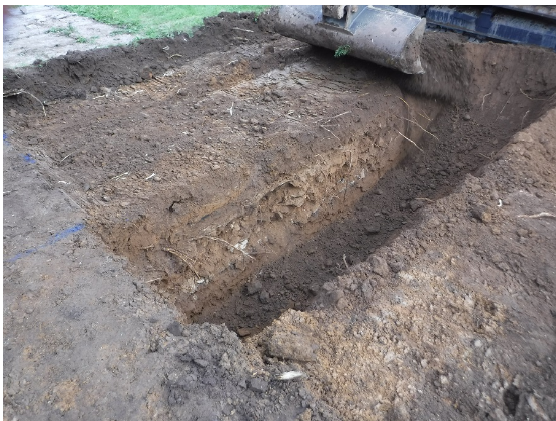
Plate 1. Northern end of the excavated area, showing stone rubble deposit (03)
