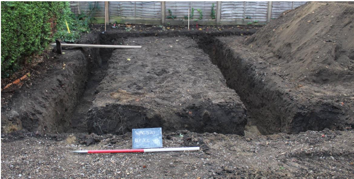
Plate 2: Completed Footings Trenches (southern extent).
