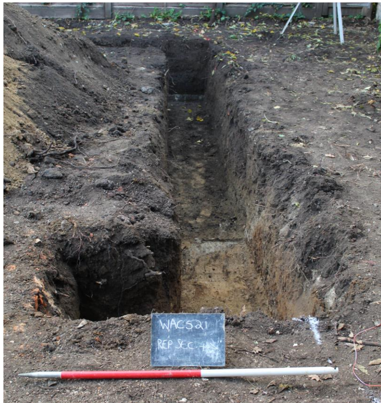
Plate 3: Completed Footings Trenches (northern extent).
