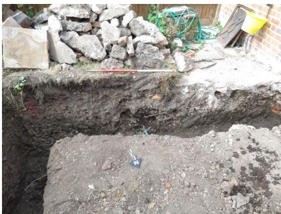
Plate 3: Sections 1 and 2, post-ex, looking south south-west.
