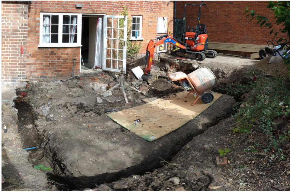
Plate 2: Area of development, post-ex panorama, looking north north-
