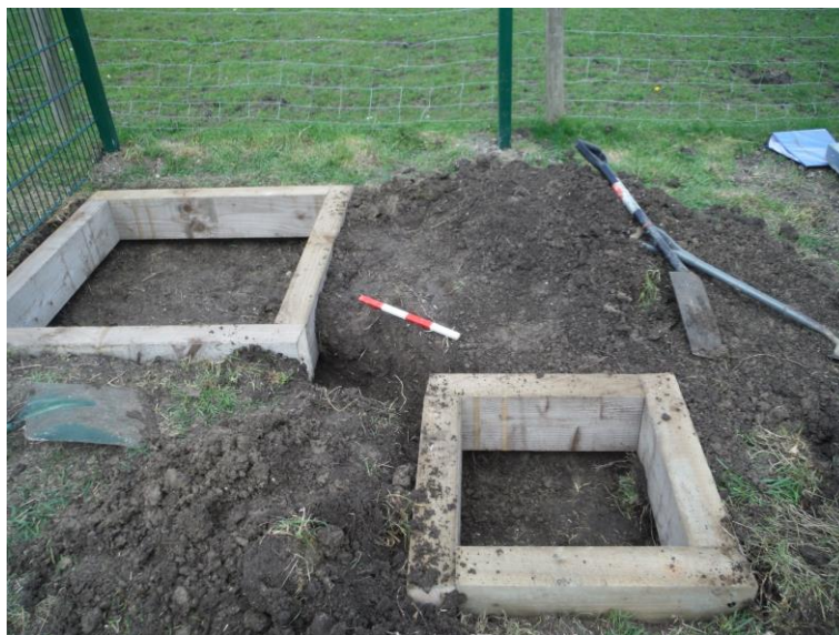
Plate 1: Location of the two concrete pads
