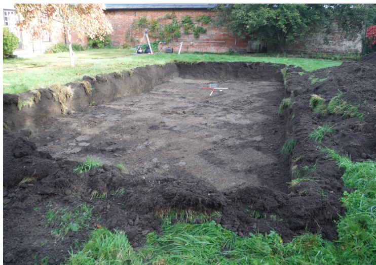
Plate 2: Pool Area Excavation
