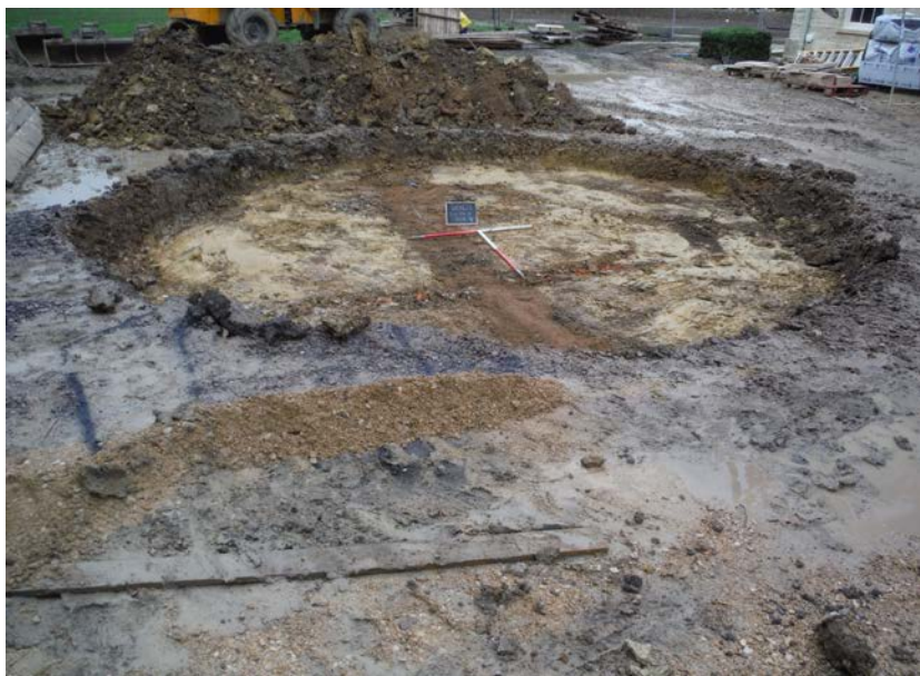
Plate 2: Post-excavation of 'Pond Area', showing service trench 32. Looking west.
