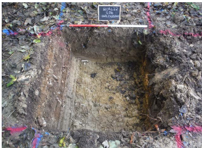
Plate 4: Section 06. Representative section of square footing trench. Looking south-west.
