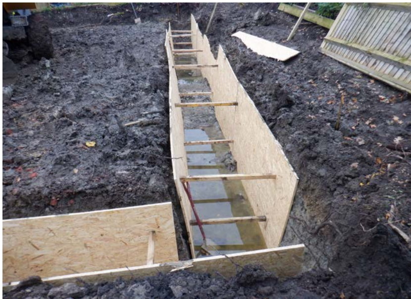
Plate 2: Shoring of trenches. Looking south-east.
