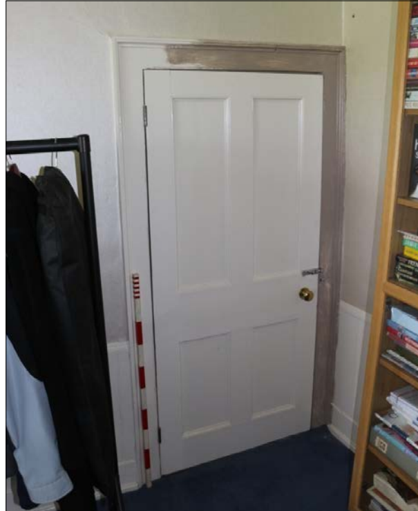
Plate 17. Room F1, four panel door to the bathroom
