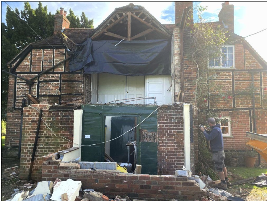
Plate 24. Demolition of lower floor structures
