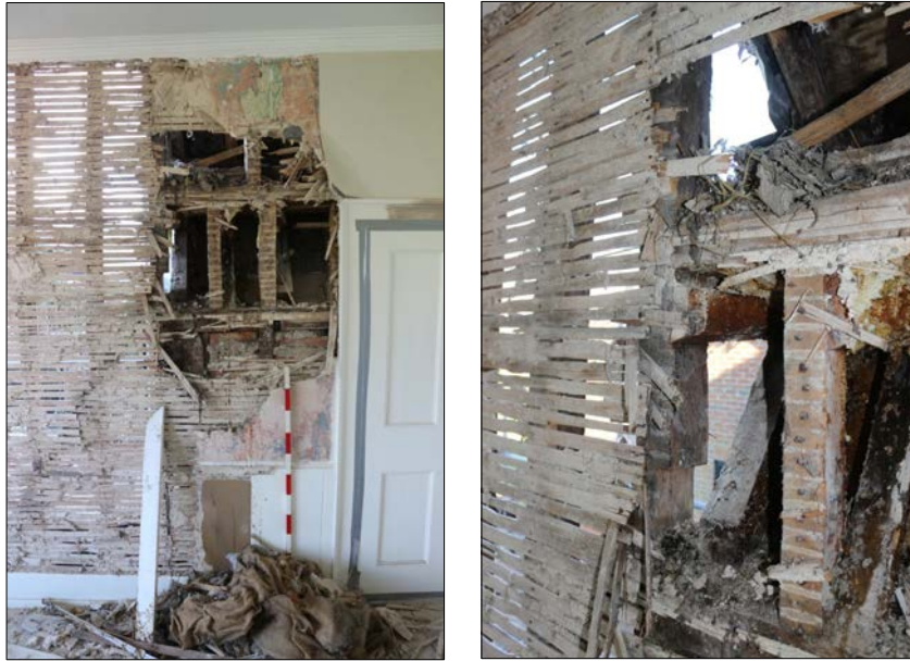
Plate 27. Intersection of the extension with the earlier building, as seen internally
