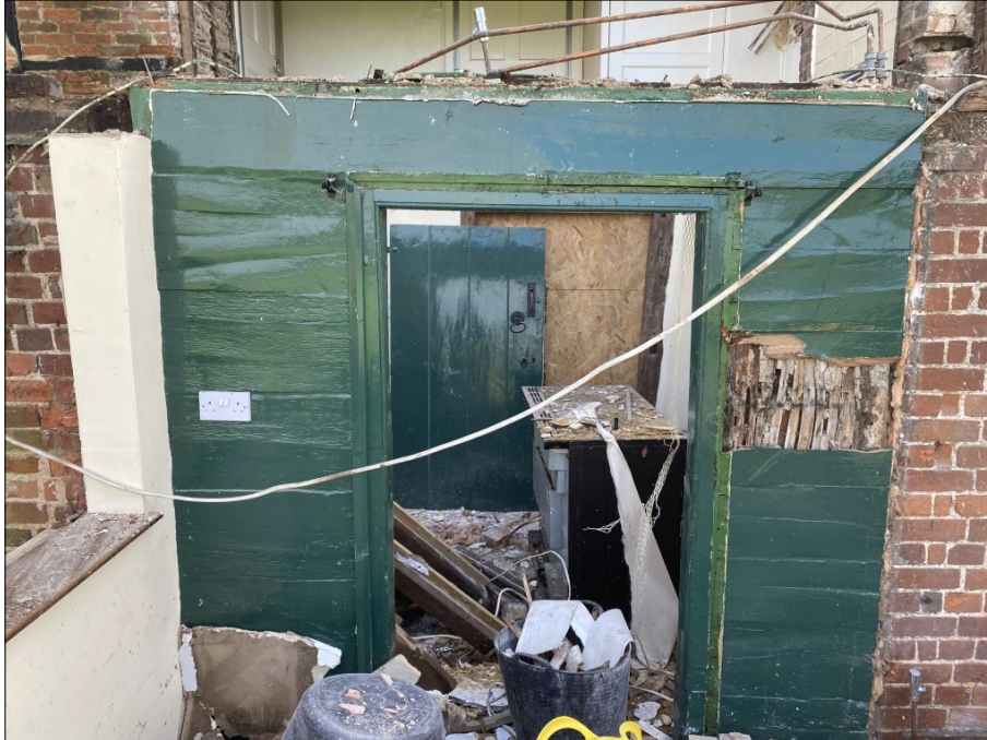
Plate 23. Rooms G1 and G2, timber panel
