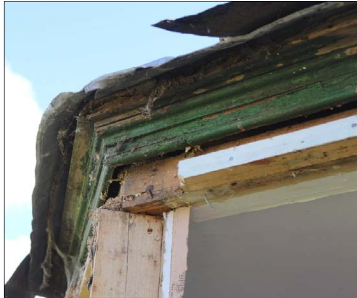
Plate 31. Earlier painted architrave at the top of the bay
