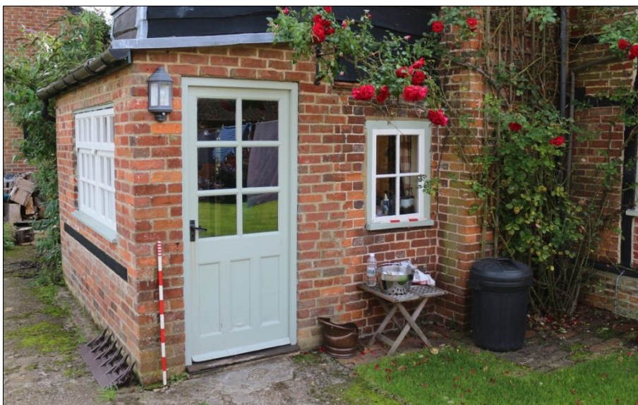
Plate 3. Lower part of the south west facing elevation,
