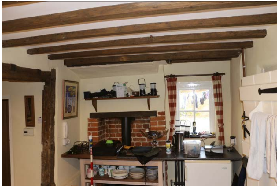
Plate 10. South west wall of Room G1 and ceiling/floor joists of F1
