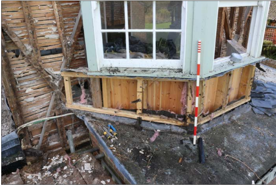
Plate 29. Modern framework of the bay window
