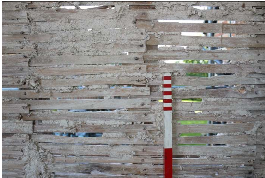
Plate 28. Room F1, Internal lath and plaster
