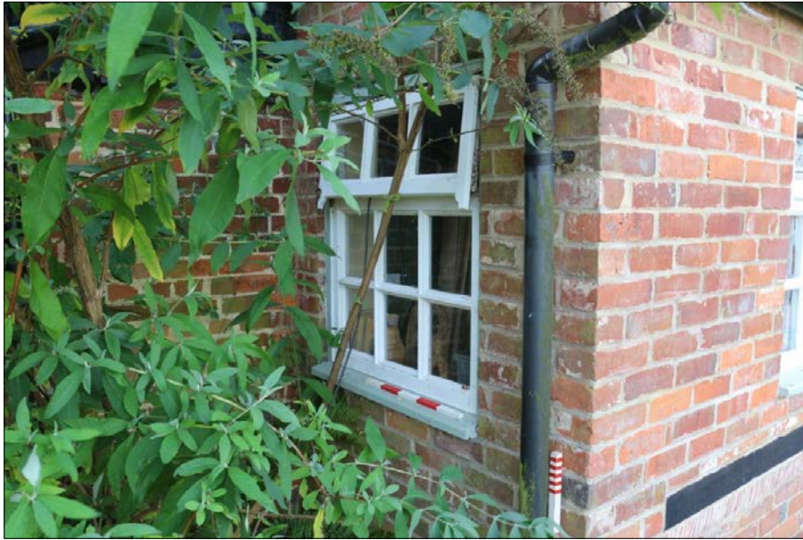
Plate 7. Window into G2 on the north east facing elevation
