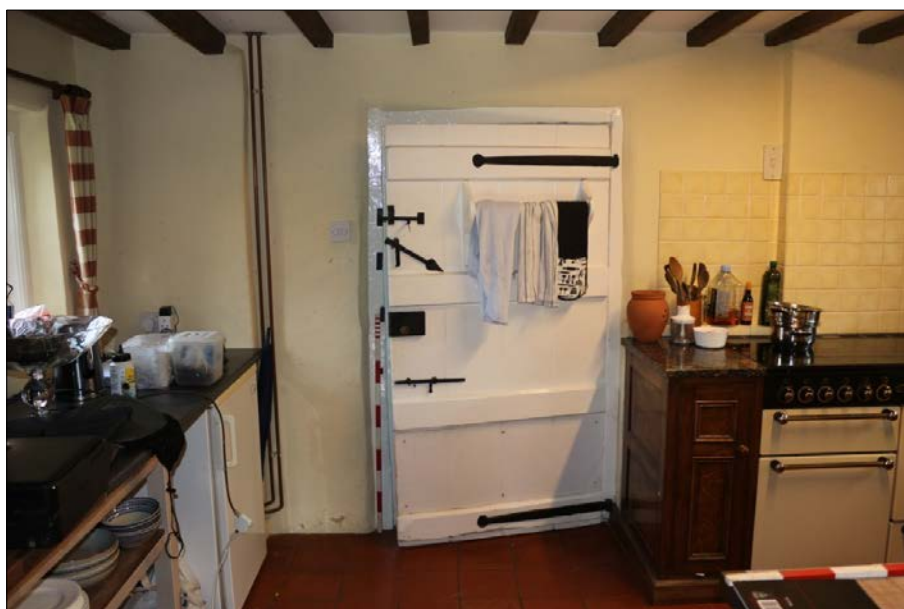
Plate 9. Historic plank door within Room G1
