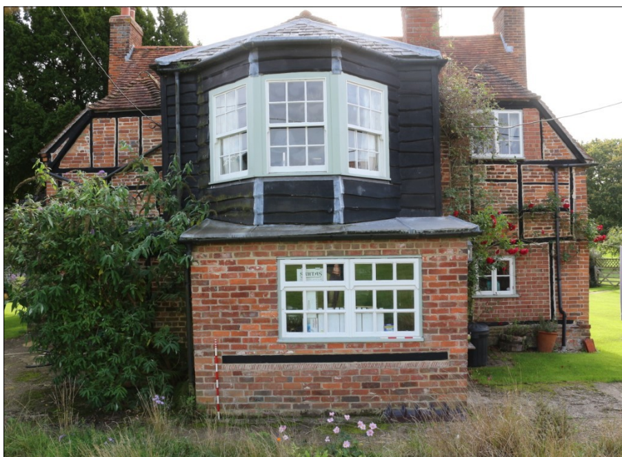
Plate 4. North west facing elevation
