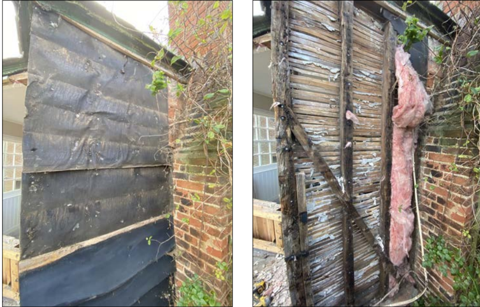
Plate 25. Removal of weatherboarding, membrane and fibre insulation
