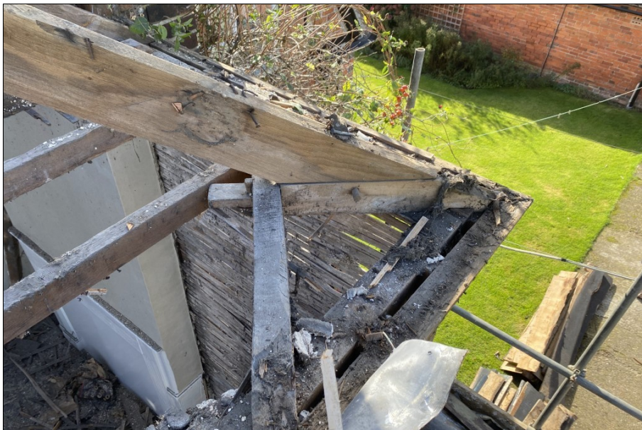
Plate 34. Corner and dragon tie-beam assembly supporting a hip rafter
