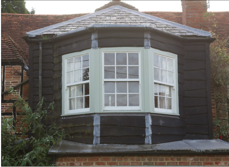
Plate 5. Bay window on the north west facing elevation
