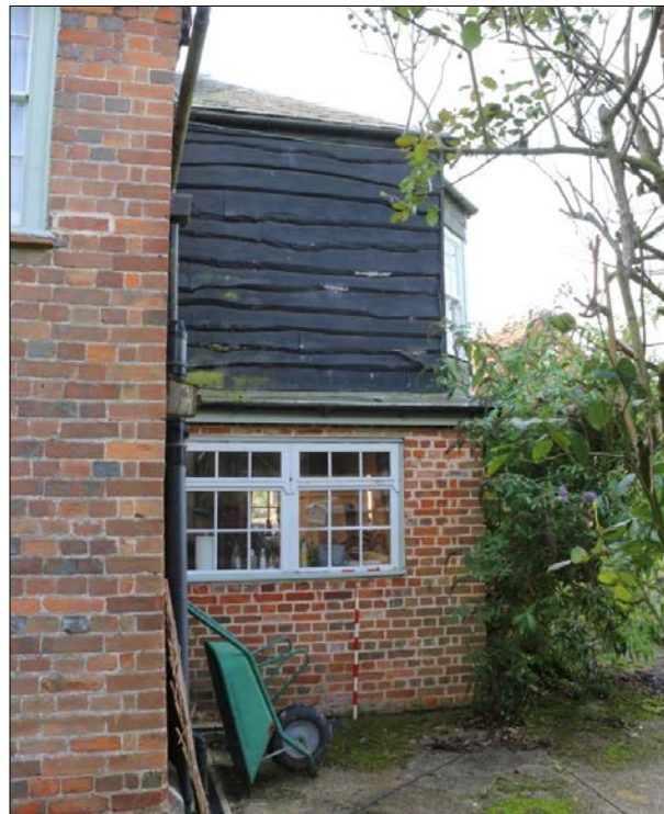
Plate 8. North east facing elevation
