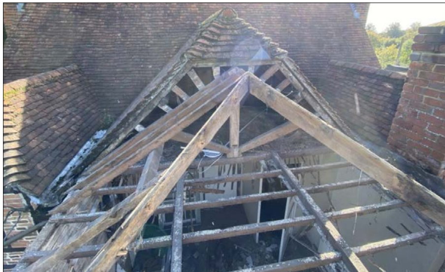
Plate 32. Roof structure of the timber framed extension
