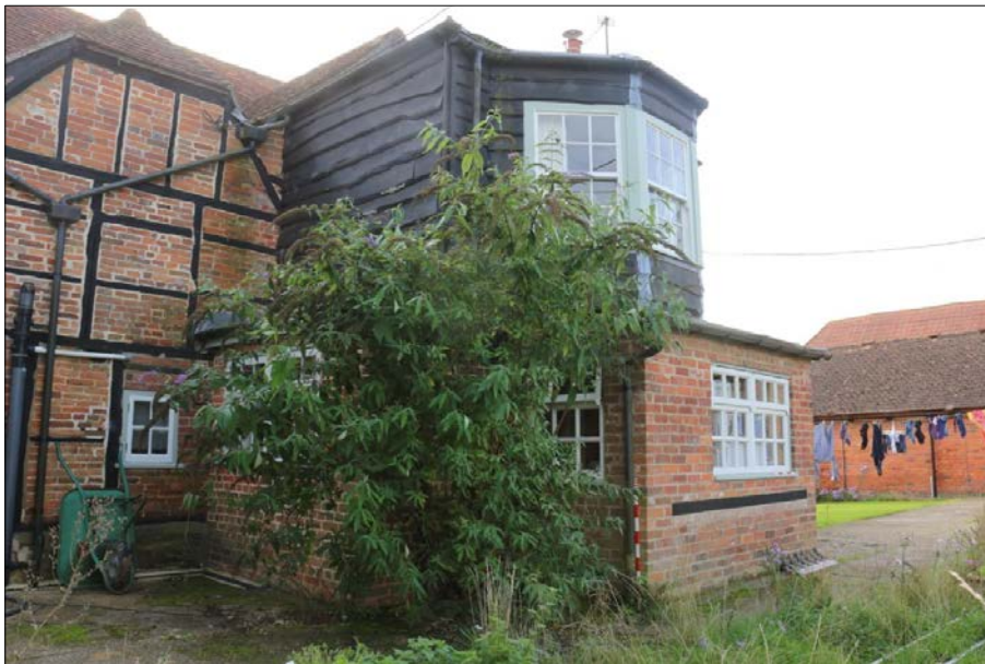
Plate 6. North east facing elevation
