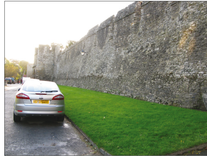
Detail of batter on city wall between Bastions 11 & 12
