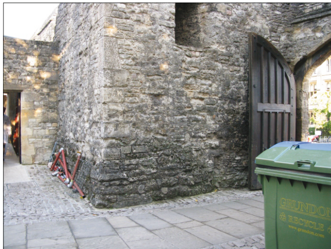
Detail of west wall Bastion 12
