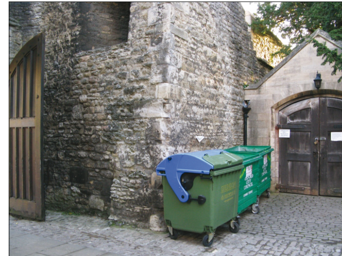
Detail of east wall Bastion 12
