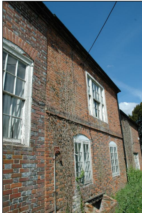
Figs 5 & 6. The East Elevation with the south end on the left and north on the right. Distortion from differential settling of the two halves is clearly visible in Fig. 3.
