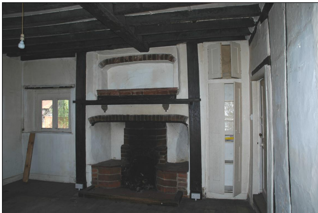
Fig 20. The north wall of the Reception Room, showing the door blocked to make a window and the fireplace. The door on the right hand wall leads to the main ground-floor corridor.
