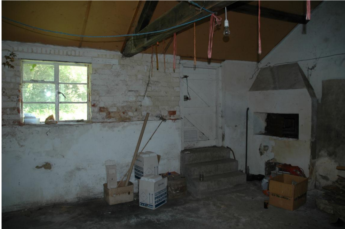
Fig 61. The south-east corner of G10, showing the eastern window and entrance and the bread oven in the south wall. The open truss ceiling is also visible.
