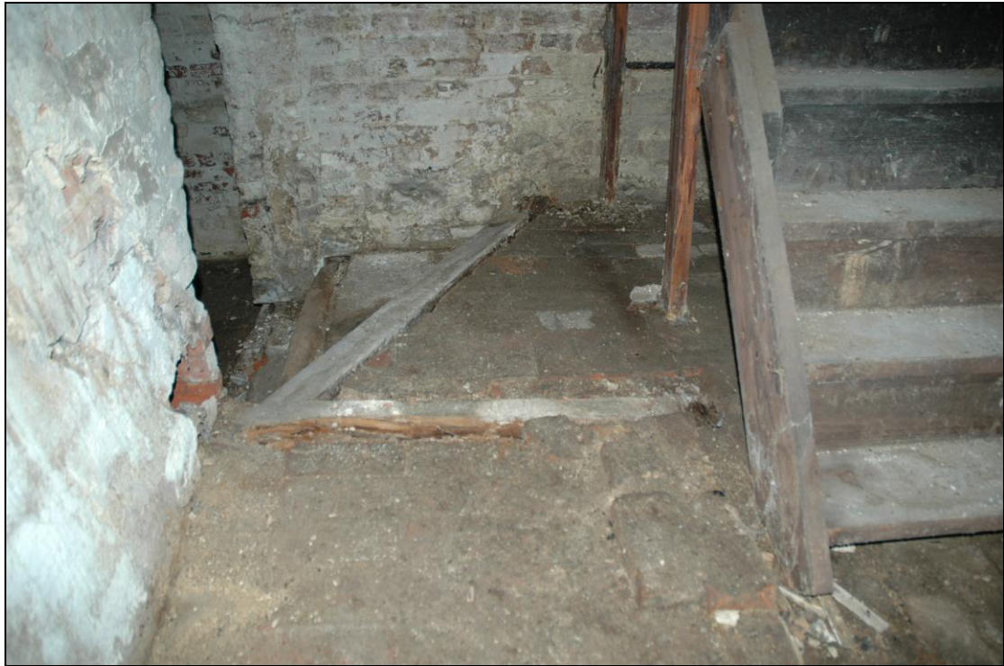
Fig 22. Present position of stair to the basement (B1), with evidence on the left hand wall of its original position with the turn in the stair to the vaulted cellars (B2 & B3) at the foot.
