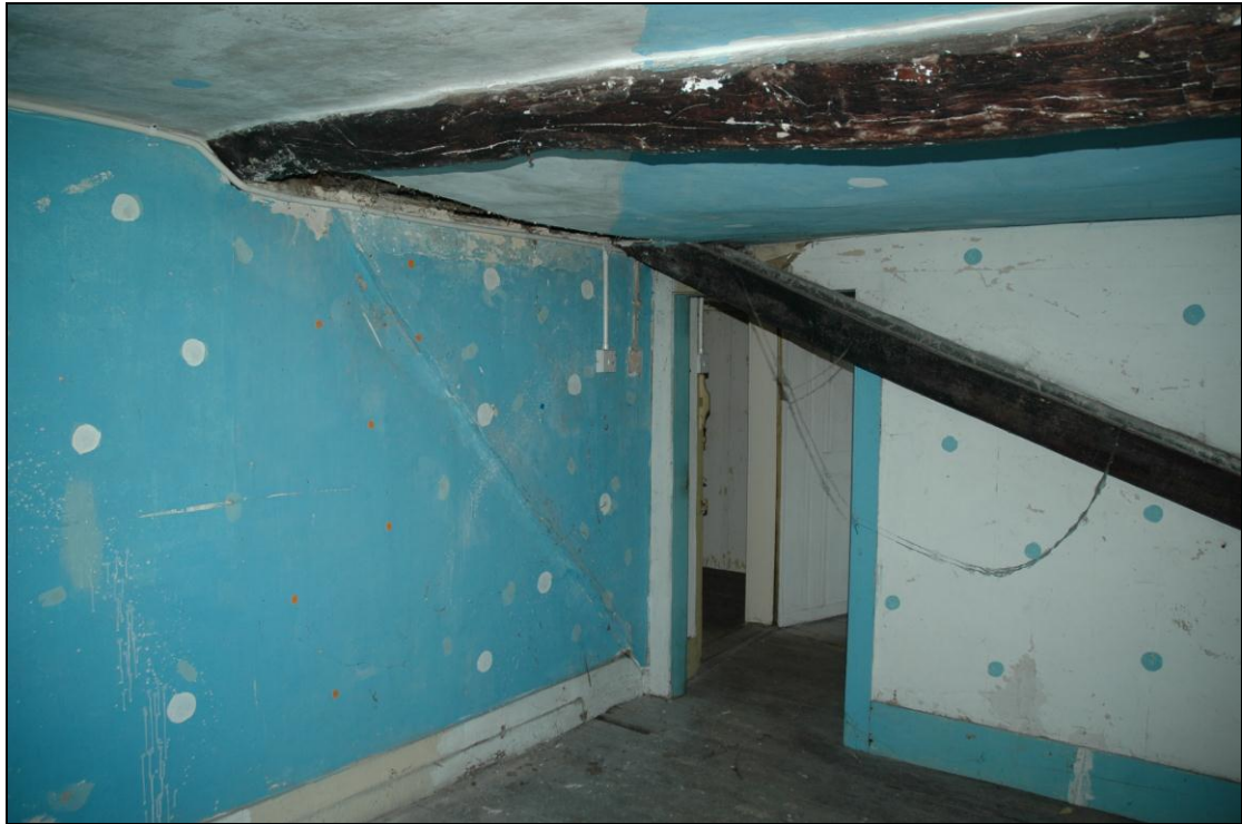
Fig 52. The south-east corner of Room S3, showing the slope of the original roof, with its purlin above and the storm water channel, which runs through the room, cutting across the door.
