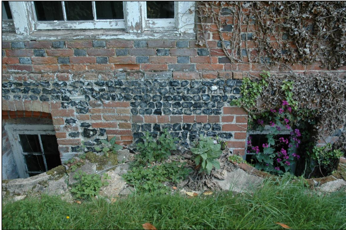
Fig 2. The brick and flint plinth of the north part of the west elevation with basement windows and light-wells
