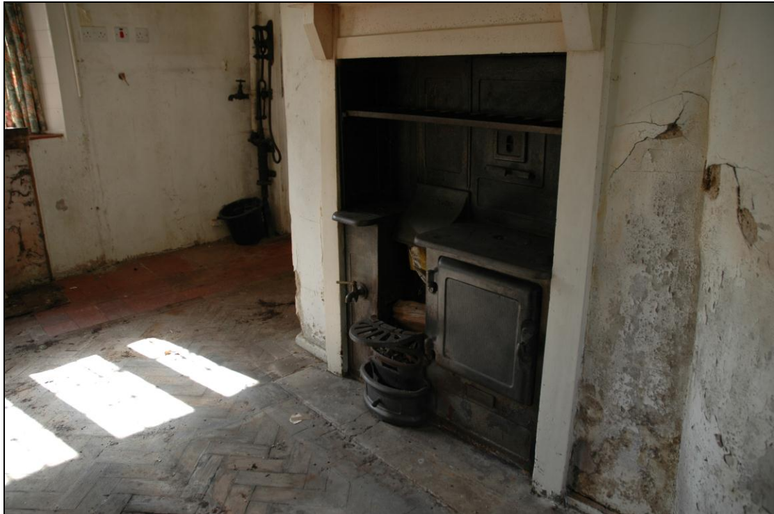
Fig 57. The kitchen range, showing also the herringbone parquet floor and the hand water pump in the corner with tile floor surround.
