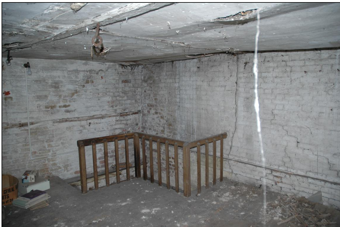
Fig 59. The south-east corner of F6, showing the head of the wooden stair. Where the rail meets the south wall is where the blocked up window of room F4 is, to the left of the crack along the straight joint. The ceiling beam in the foreground shows the hooks.
