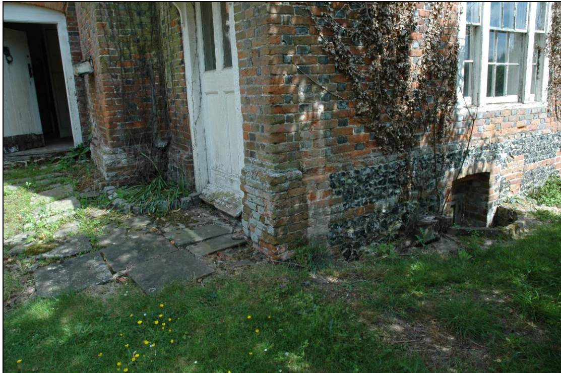
Fig 13. The north-west corner of the main house, showing the different elements of the plinth. Also seen here is the present farmhouse entrance in the first extension and some early paving slabs. The rest of this yard appears to have been paved with pebbles, which would have aided drainage and is often found in courtyards of the late 17 th century. Much of this has now overgrown with grass.
