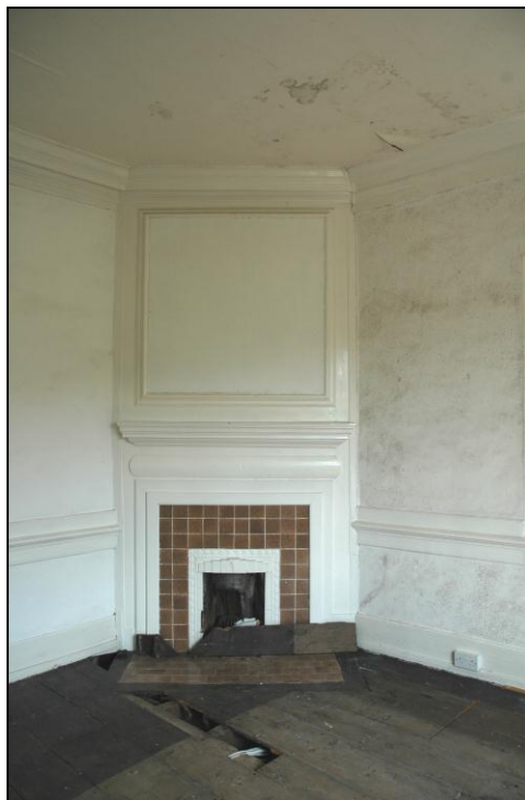
Fig 48. The corner fireplace in Bedroom F4. Just at the right edge of the photograph can be seen the recess of the blocked north window.
