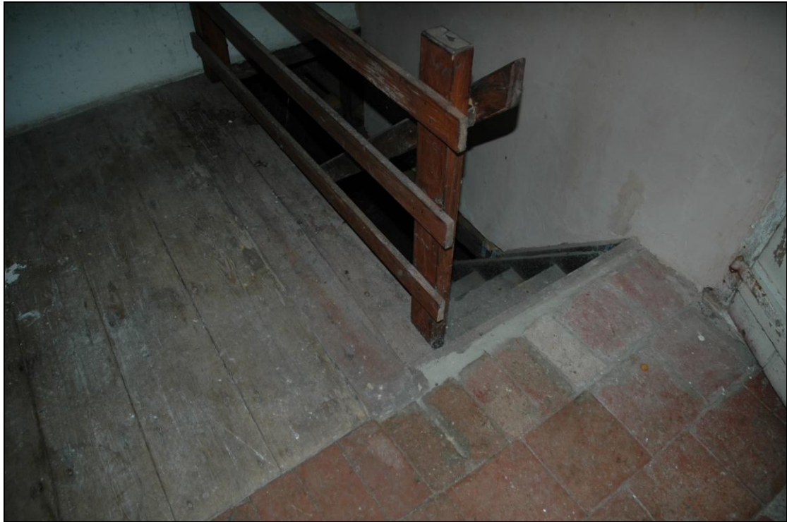
Fig 27. The north side of the floor of the dairy/larder, showing the difference between the tiled floor on the south side and the timber floor on the north and the present cellar stair cut through the latter.
