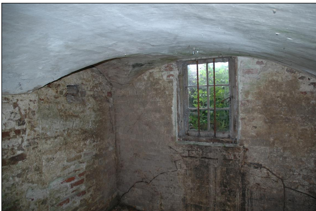
Fig 25. The east end of Basement B3, showing blocked door to the left (north) and the barred side-hung casement window at the east end.
