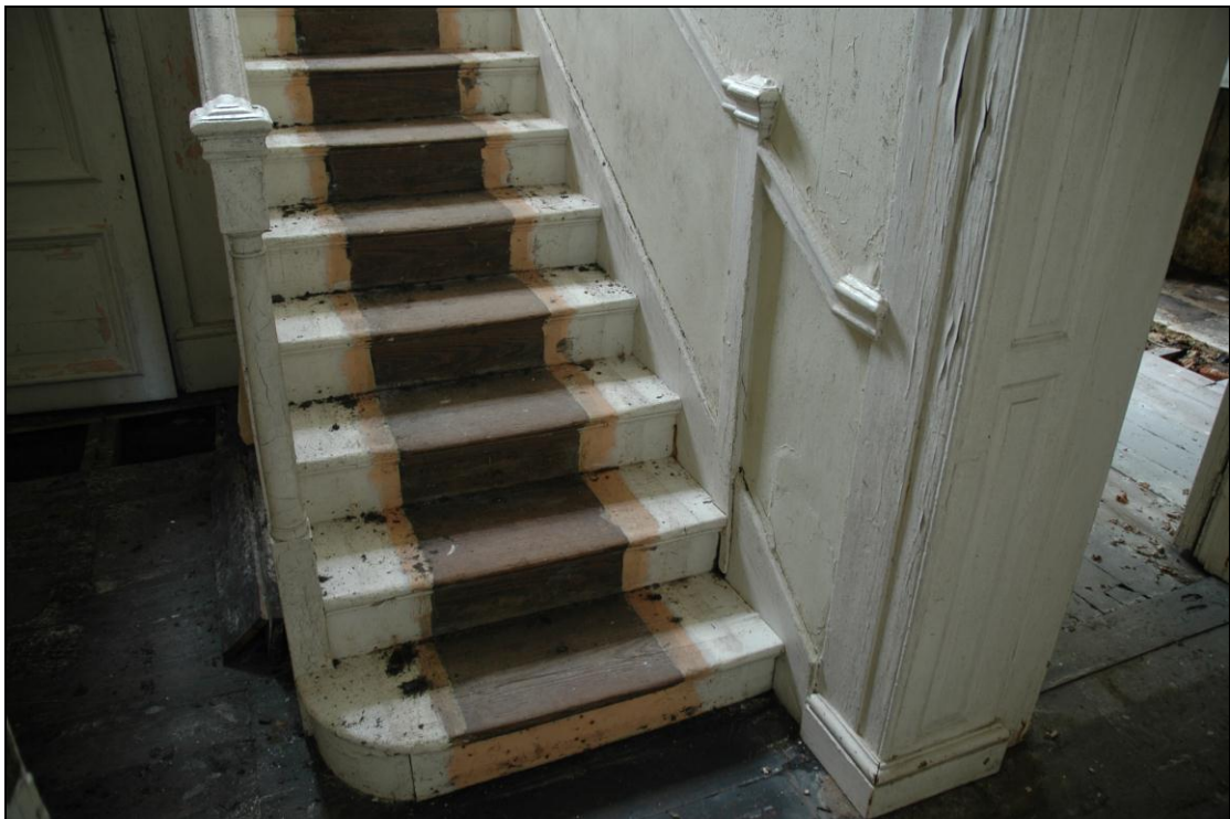
Figs 28 & 29. The Stair with turned newels and balusters with dado and pilasters.
