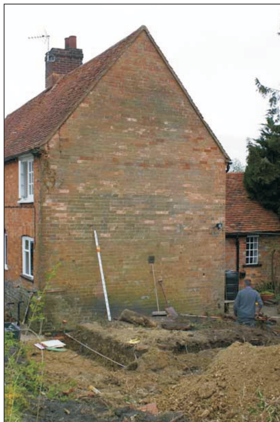
Figure 5. South-east wall of kitchen
