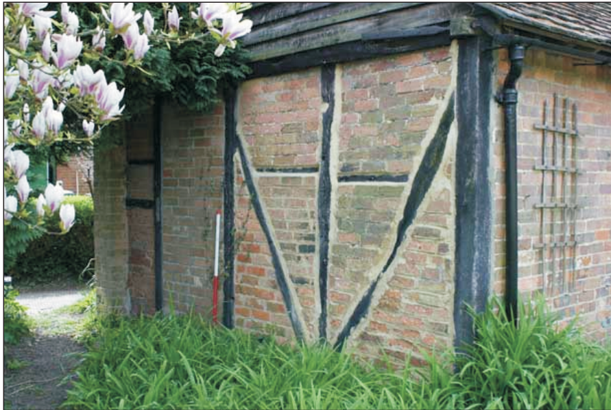
Figure 4. North-east wall of store
