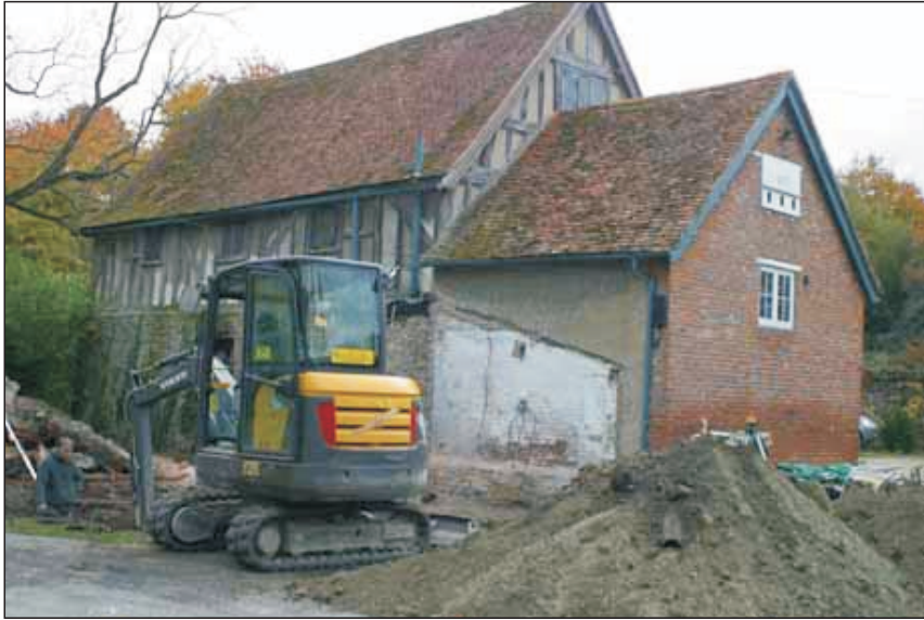
Plate 1. South-west facing working shot of the Guest House
